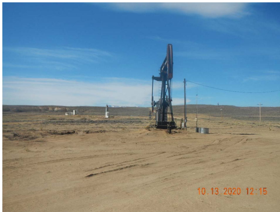
Photo 1. Overview of location taken at entrance facing west. Freshly disturbed soil with no stormwater controls.
