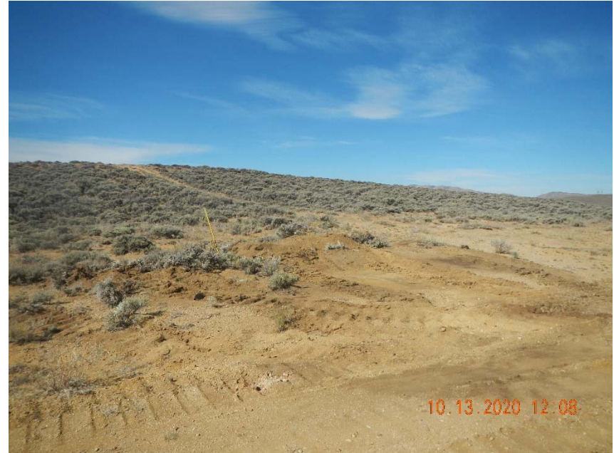
Photo 2. Freshly disturbed soil with no stormwater controls.
