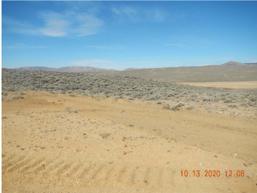
Photo 3. Freshly disturbed soil with no stormwater controls.
