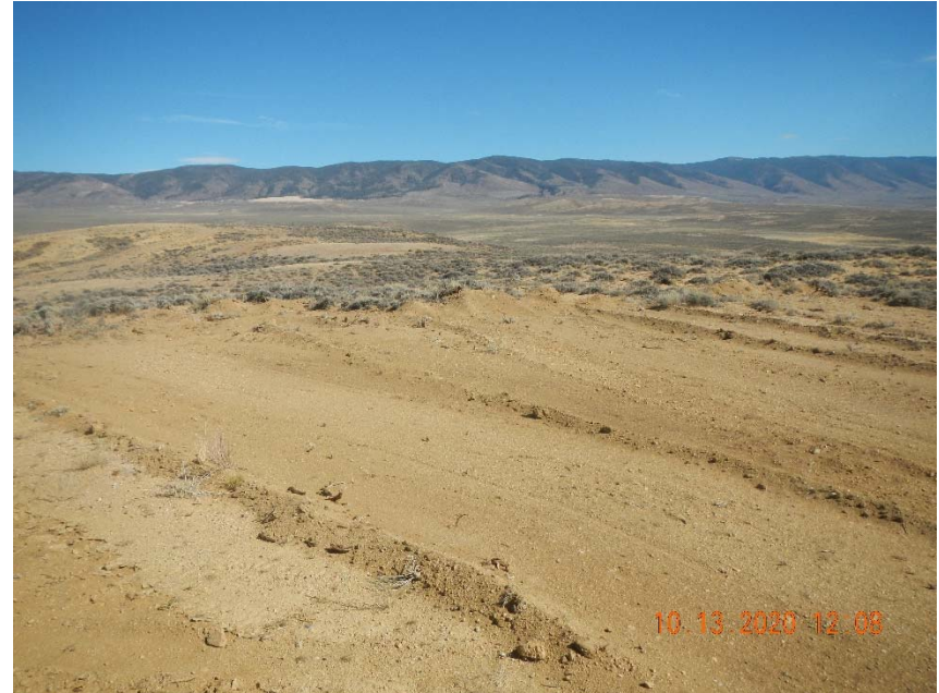
Photo 4. Freshly disturbed soil with no stormwater controls.
