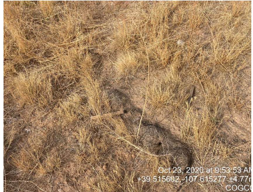
Old waddle at bottom of ditch failing
