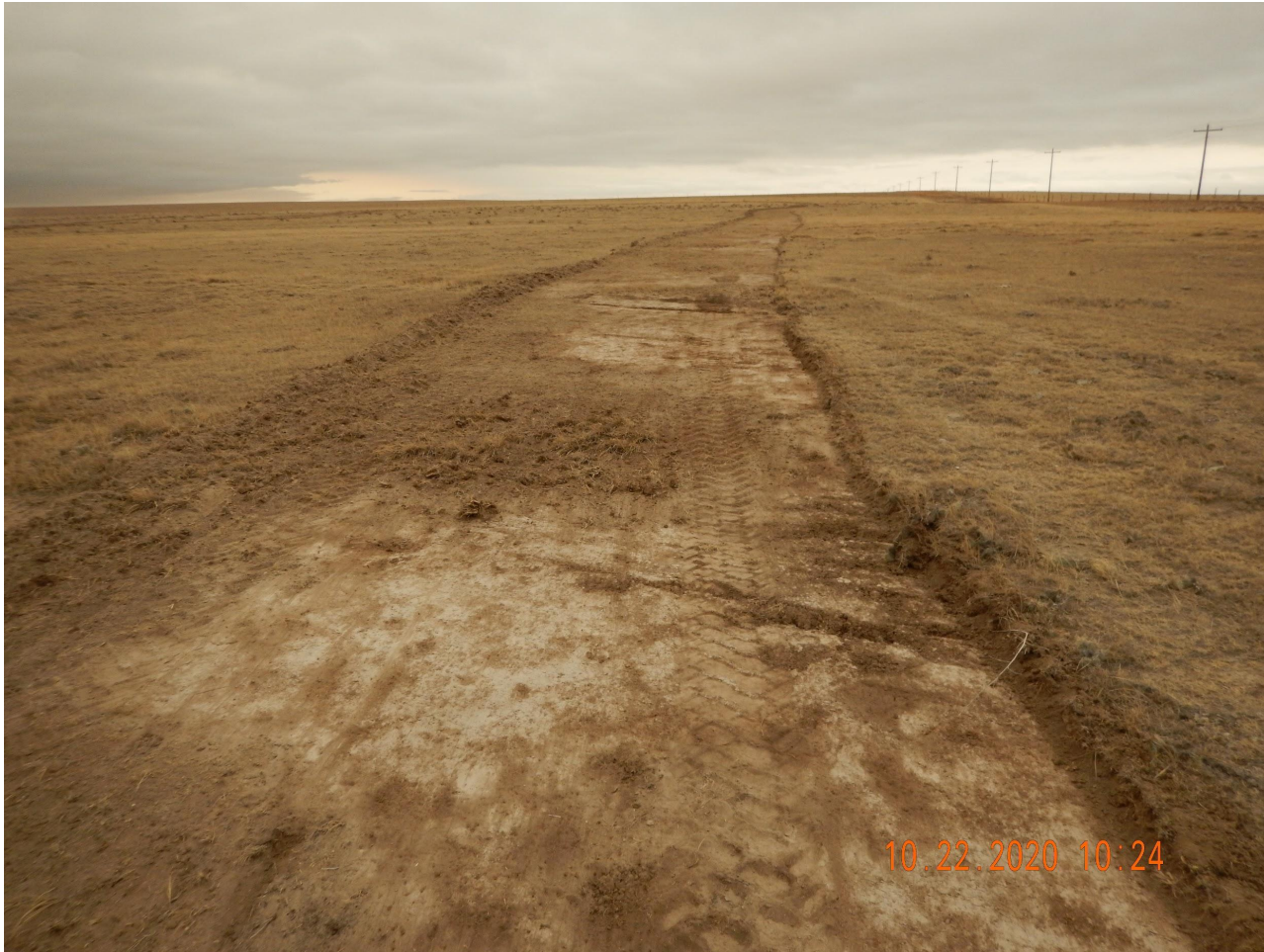
Photo 3. Photo taken from the northeastern location, facing West. Photo illustrates the Operator has failed to install stormwater BMPs prior to starting topsoil salvage operations.
