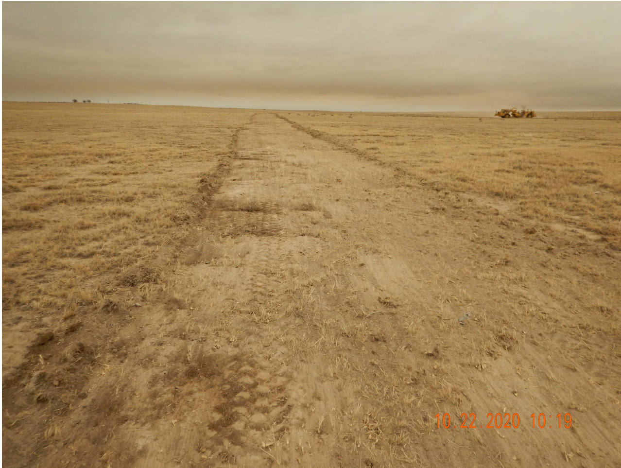
Photo 2. Photo taken from the eastern location, facing South. Photo illustrates the Operator has failed to install stormwater BMPs prior to starting topsoil salvage operations.
