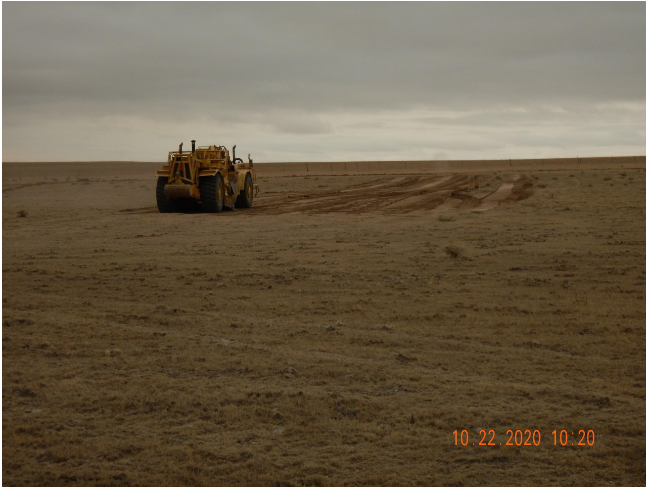
Photo 1. Photo taken from the eastern location, facing West. Photo illustrates the Operator is in process of salvaging topsoil. However, Operator has failed to install stormwater BMPs prior to starting topsoil salvage operations.
