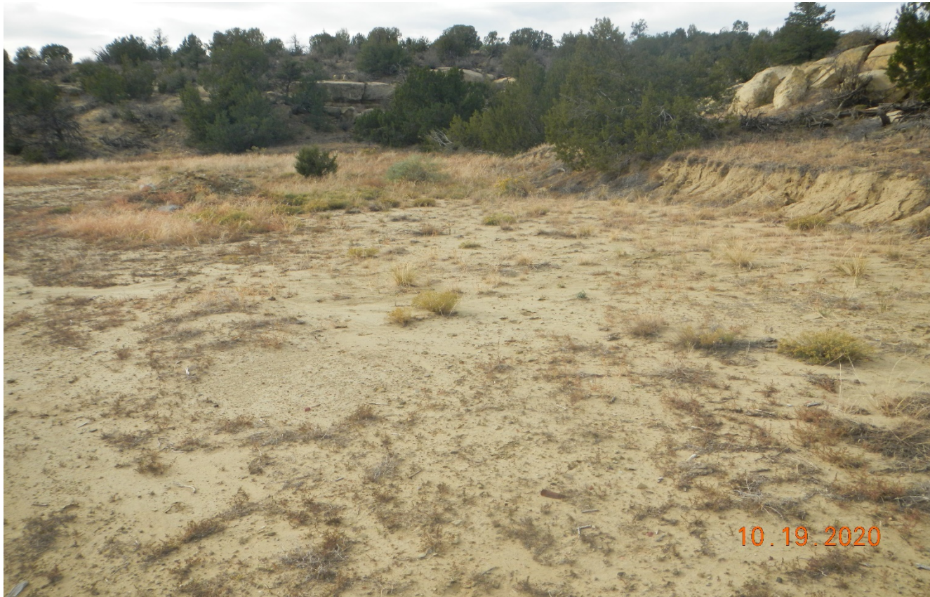
Photo 3. Facing southwest at the location. The cut slope is shown in the right side of the o. The location will need to be recontoured and reclaimed.
