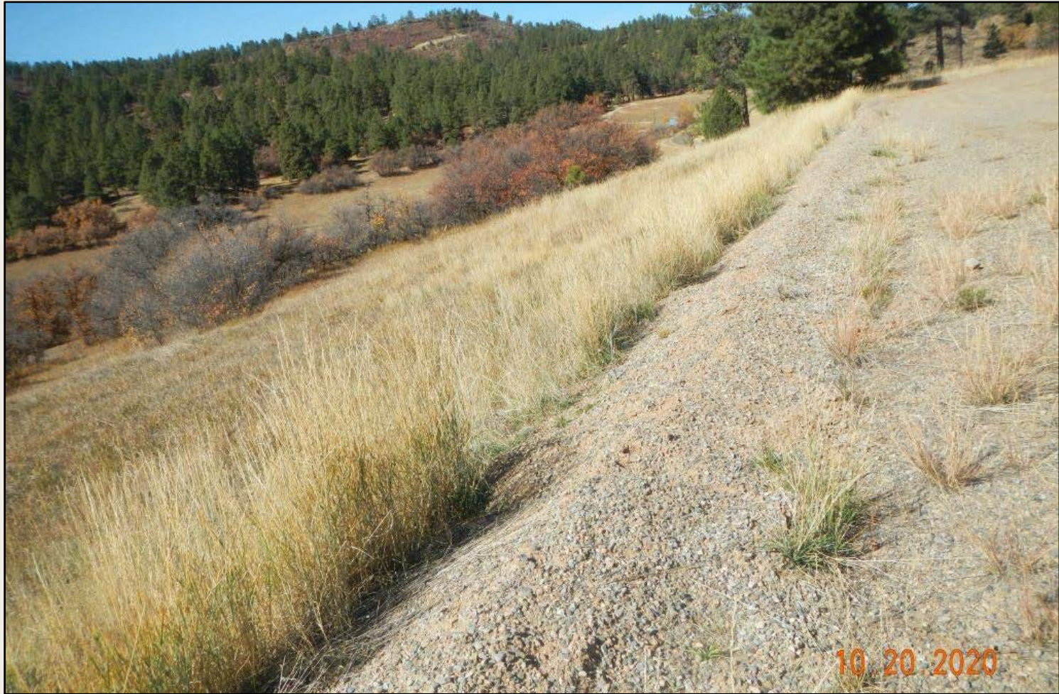
Photo 2. View of the southern fill slope from the southeastern corner facing westward. Revegetation is progressing with western wheatgrass, sand dropseed, and smooth brome.
