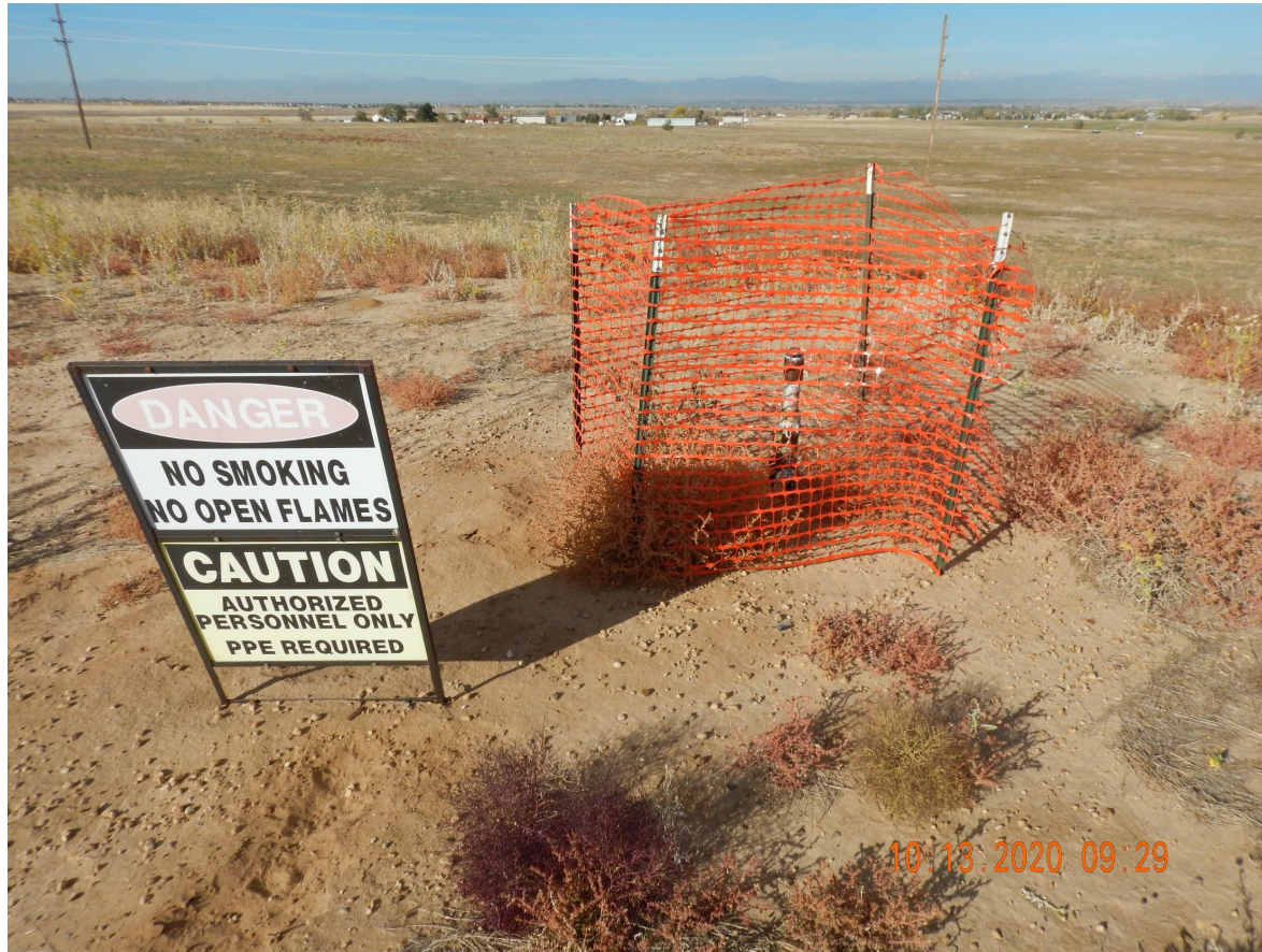
Photo 1. Photo taken from the western location, facing West. Photo illustrates the Operator has failed to remove all equipment (i.e, riser).
