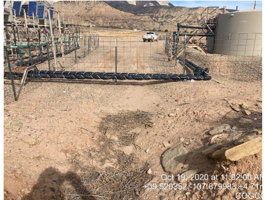
BMP's require maintenance(sediment traps, evidence of run off)
