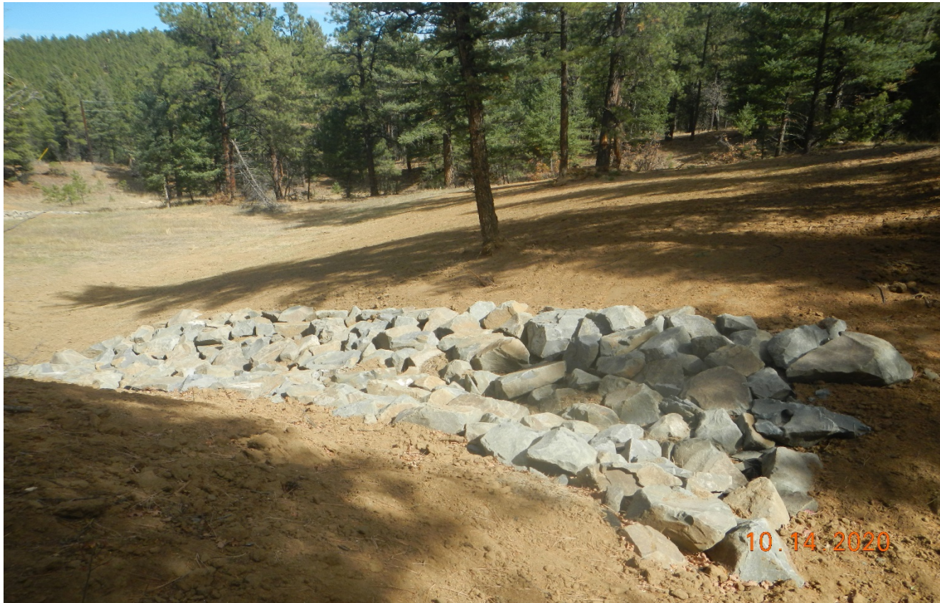
Photo 7. There is a rock riprap swale installed at the south side of the location.
