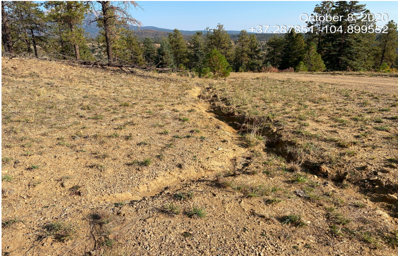
Photo 4. There is an erosion channel that is directed down toward the road from the location. This area needs to be repaired and stabilized.
