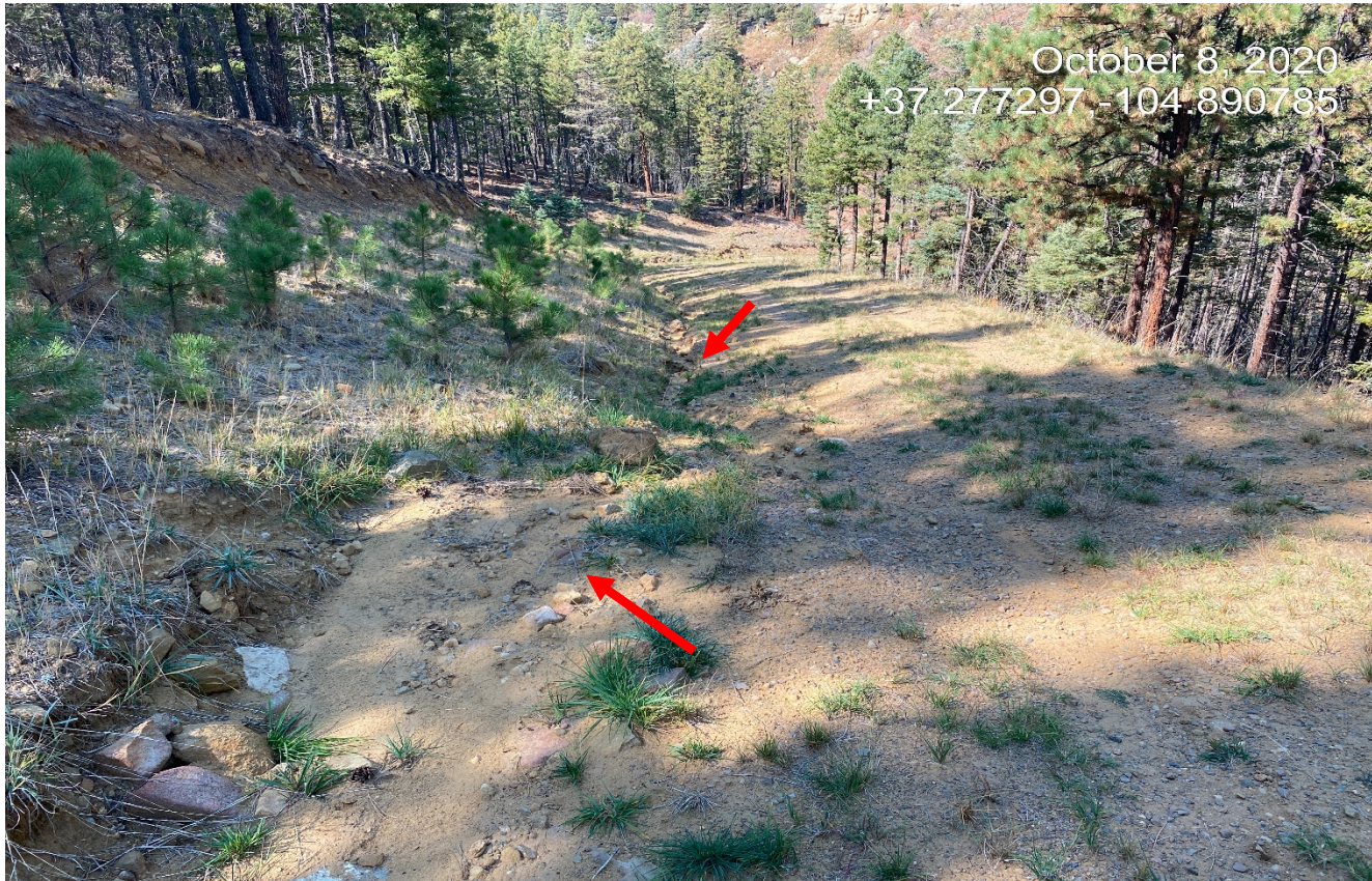
Photo 2. The culvert along the access road is filled in with sediment causing erosion down the road side.
