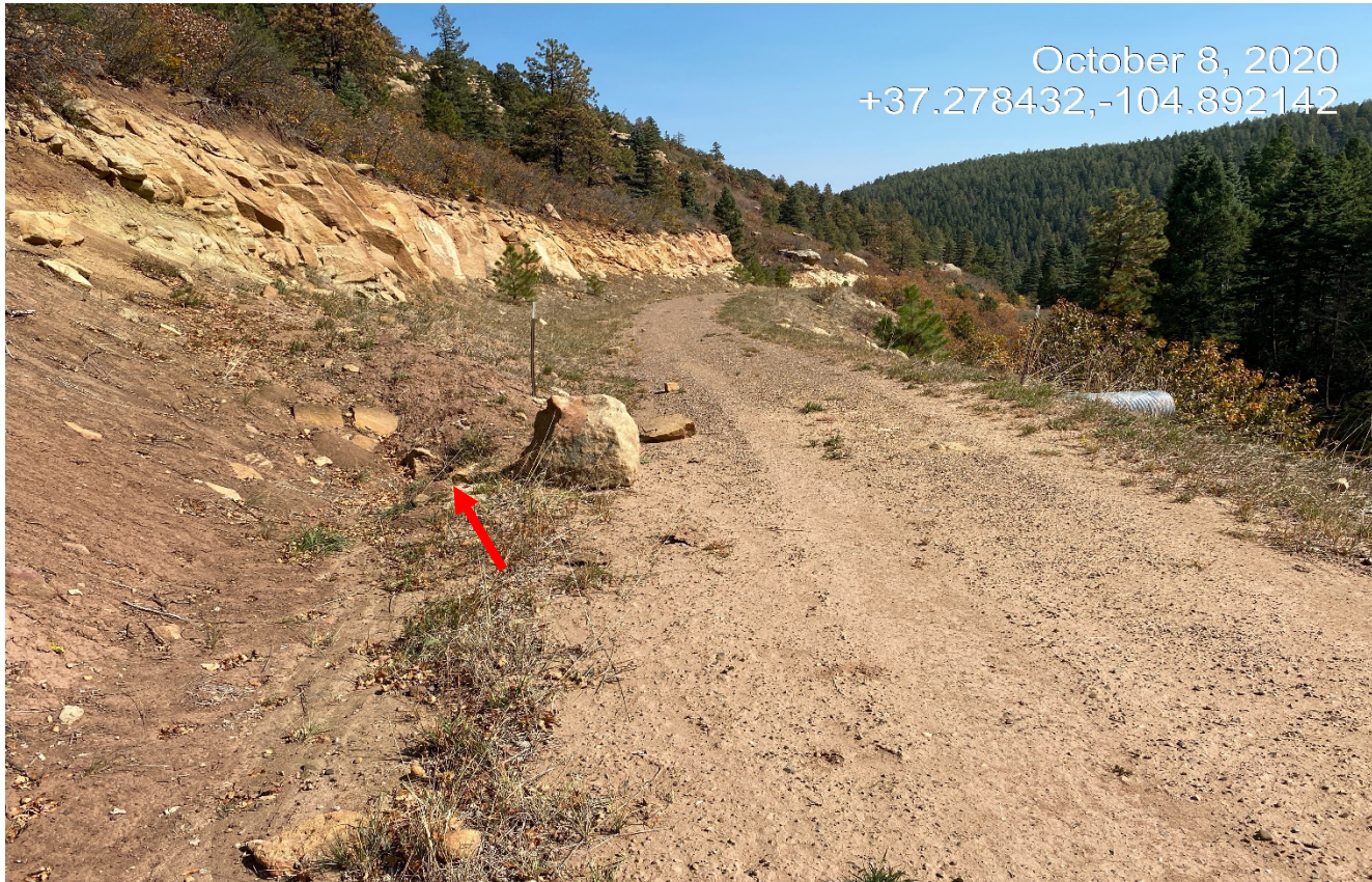
Photo 5. Facing northeast along the access road. The culvert is filled in with sediment shown at red arrow. Rocks have fallen on the road.
