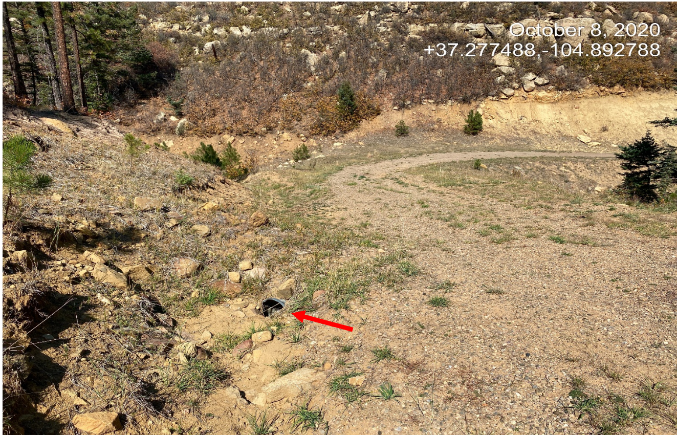
Photo 3. The road crosses the canyon bottom which creates a dam across the canyon. The culvert is filled in with sediment shown at red arrow.
