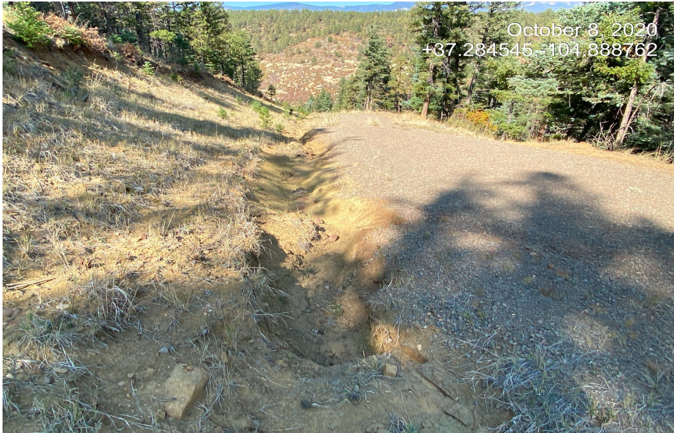
Photo 6. There is erosion occurring along the side of the road and culverts are filled in with sediment.
