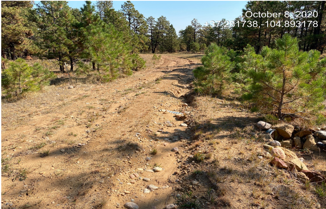
Photo 3. Stormwater is not properly diverted to the culverts along the road.
