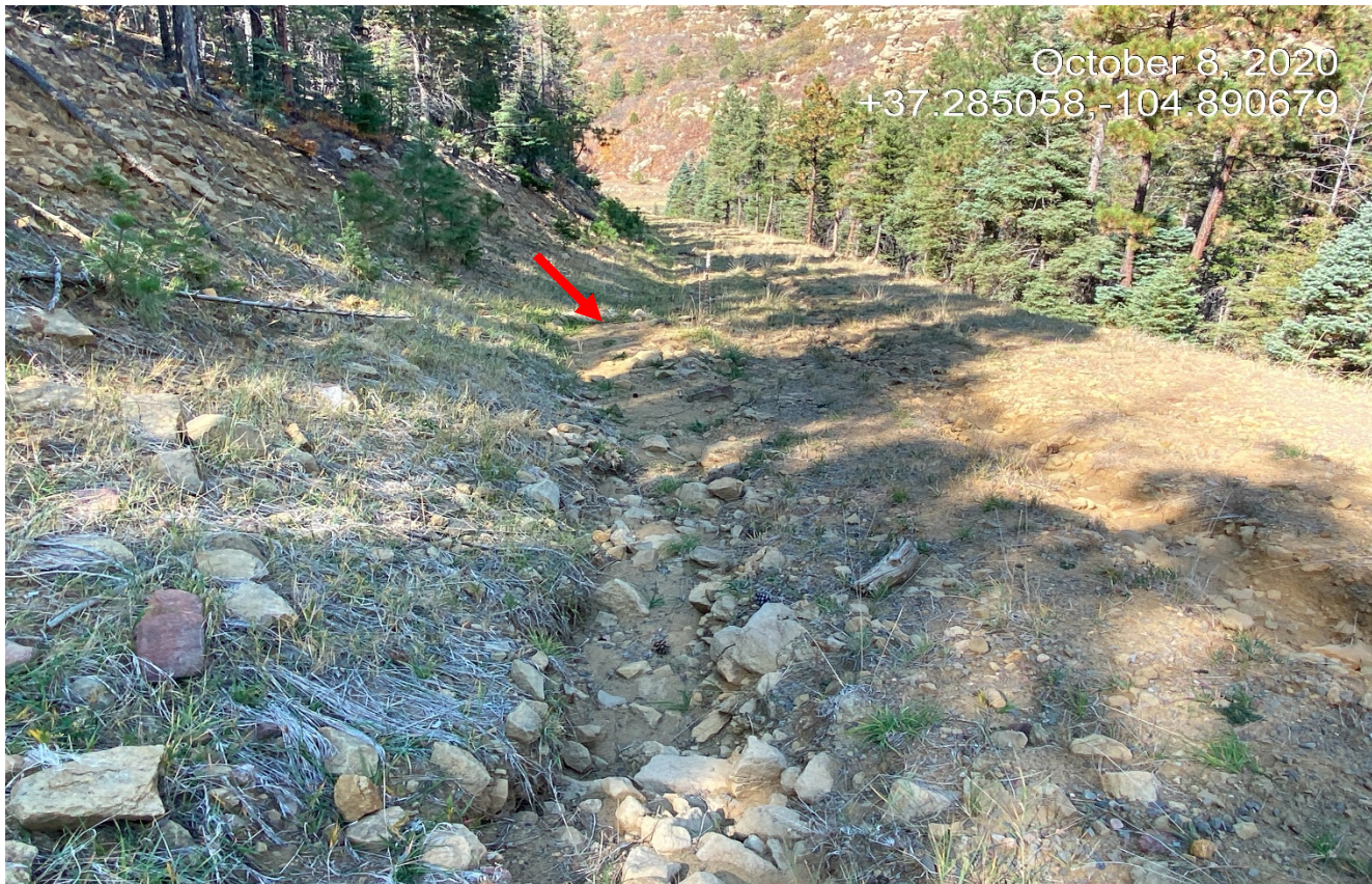
Photo 8. The arrow points to a culvert which is filled in with sediment.
