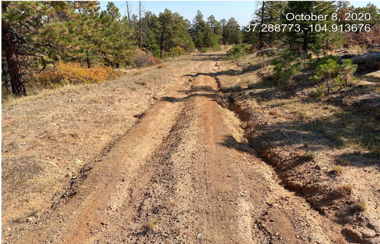
Photo 2. Facing northeast further along the access road. The road is not stabilized and there is erosion channels along the road.
