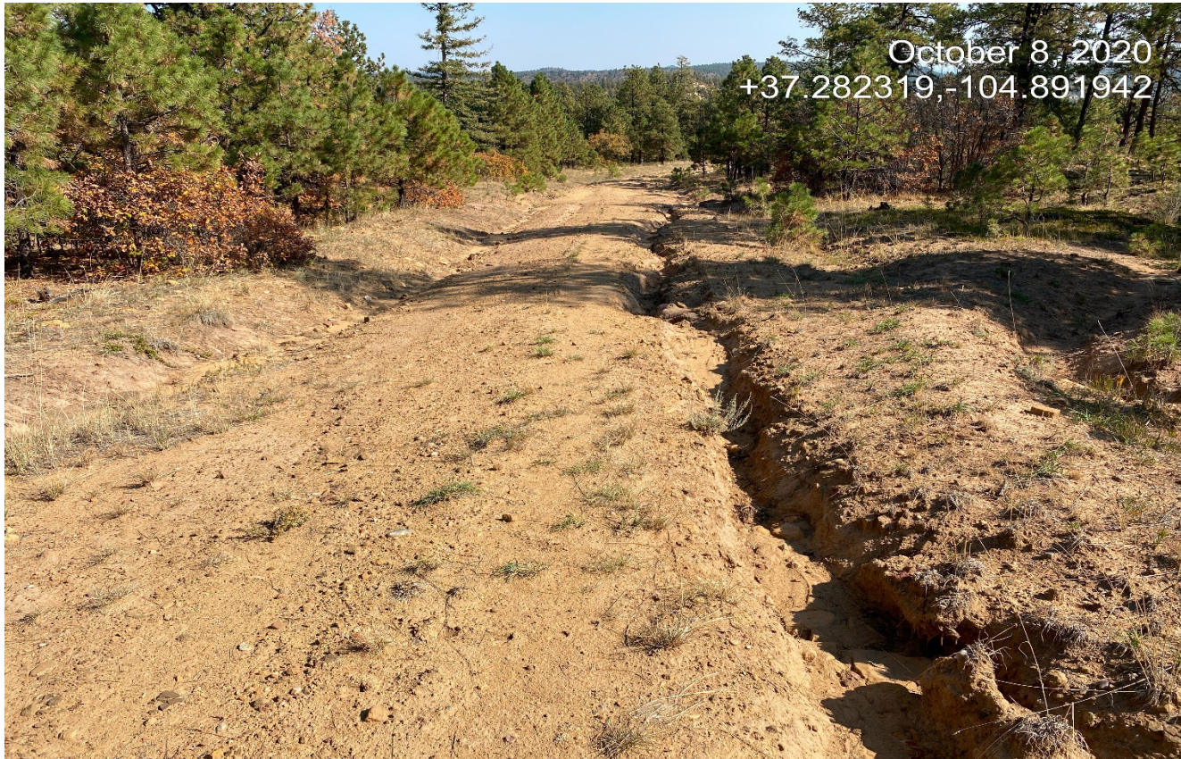
Photo 4. Facing northeast further along the access road. The road is not stabilized and there is erosion channels along the road.
