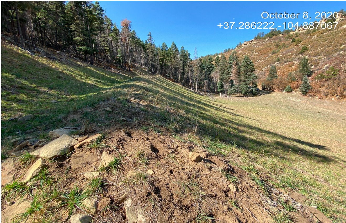
Photo 14. Facing west toward the location. There is a berm along the top portion. The berm has increased the steepness of the slope. Large berms and terracing do not match the contours of the terrain.
