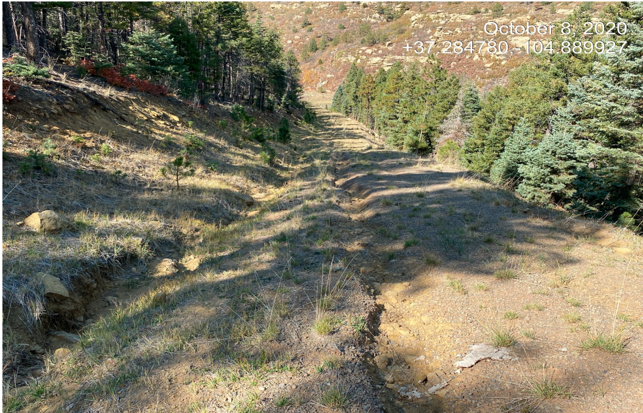
Photo 7. Facing northwest along the access road descending into the canyon. There is erosion along the road all the way down to the canyon bottom.
