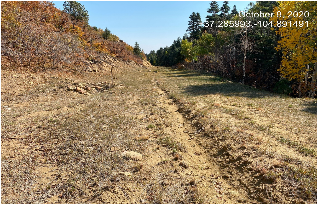
Photo 11. Facing east along the access road. It appears erosion has occurred along the road and stormwater is not diverted toward the culvert.
