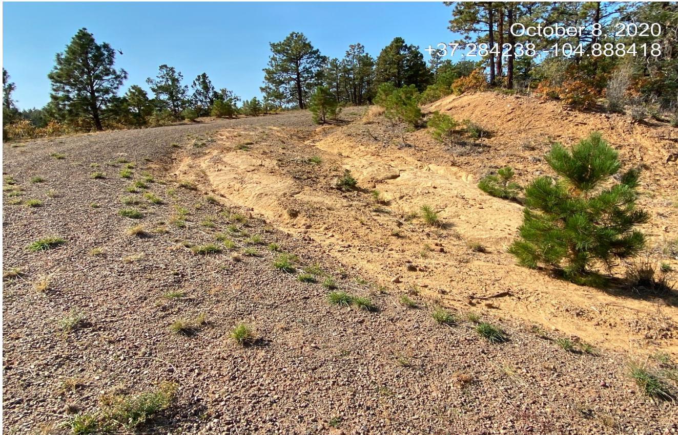
Photo 5. Facing back where the road turns down the hill side into the canyon. The side of the road is not stabilized in this area.
