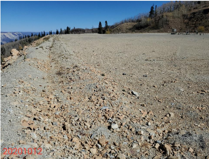
Photo 3: Photo taken from the southwest end of the Location, facing north. Photo shows overview of the Location. Photo shows interim reclamation pursuant to 1003.b has not been conducted on the Location.
