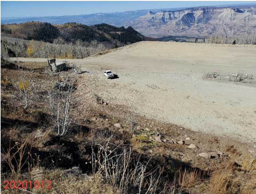
Photo 1: Photo taken from the east end of the Location, facing southwest. Photo shows overview of the Location. Photo shows interim reclamation pursuant to 1003.b has not been conducted on the Location.
