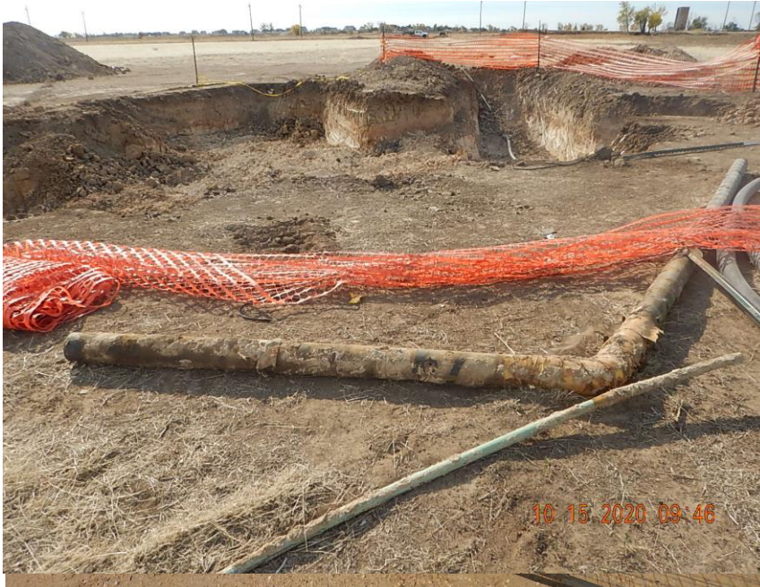
View of excavation at spill release point #465402. Looking South; Compromised section of the old flowline has been cut out and removed.
