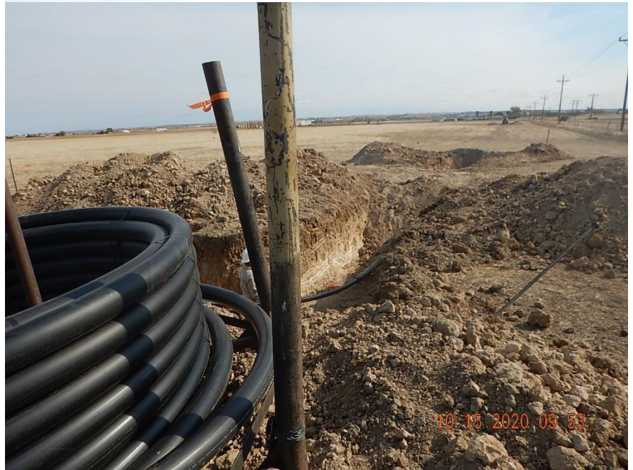
View of SW most excavation; Looking east; New 3" HDPE pipe is being pulled inside the old 4" CS flowline.
