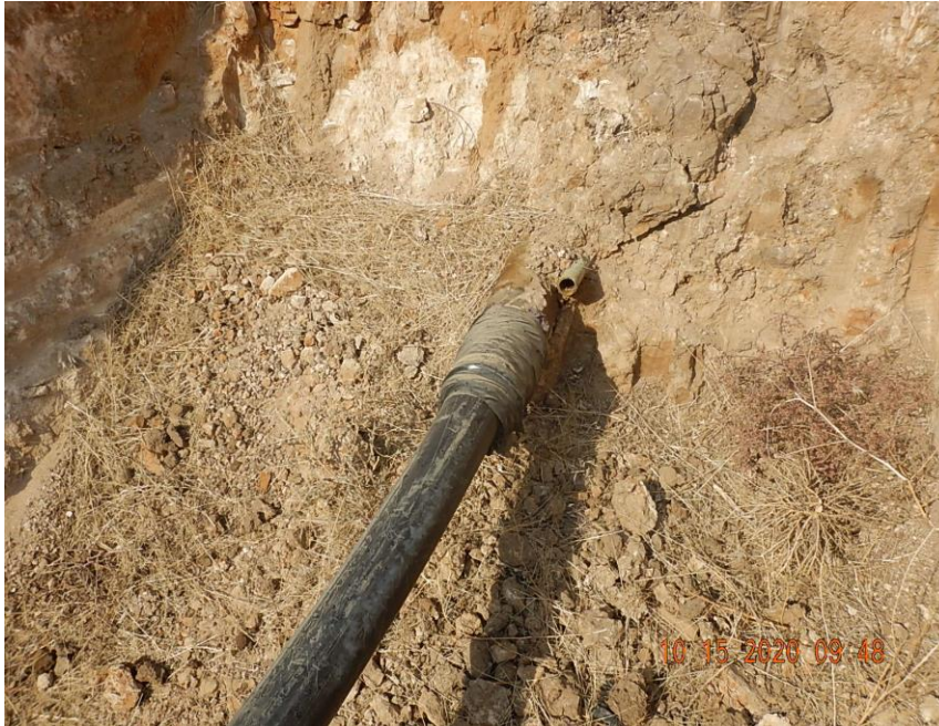
View of 3" HDPE pipe slipline replacement pipe (taped) and the cut end of the out of service 1" CS gas supply line.
