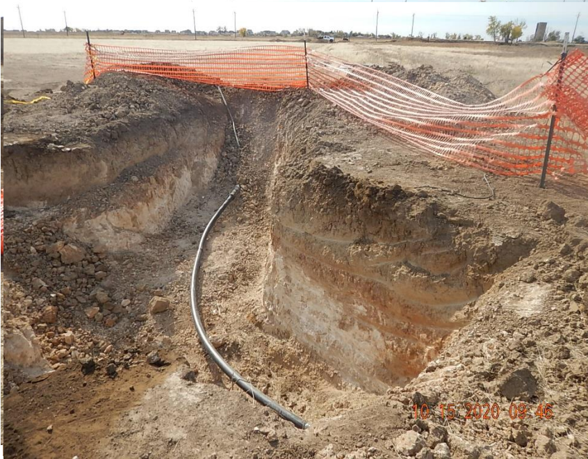
View of excavation at spill release point #465402. Looking South; New 3" SDR 11 HDPE pipe has been stung/ sliplied inside the cut end of the old 4" Consolidation flowline.
