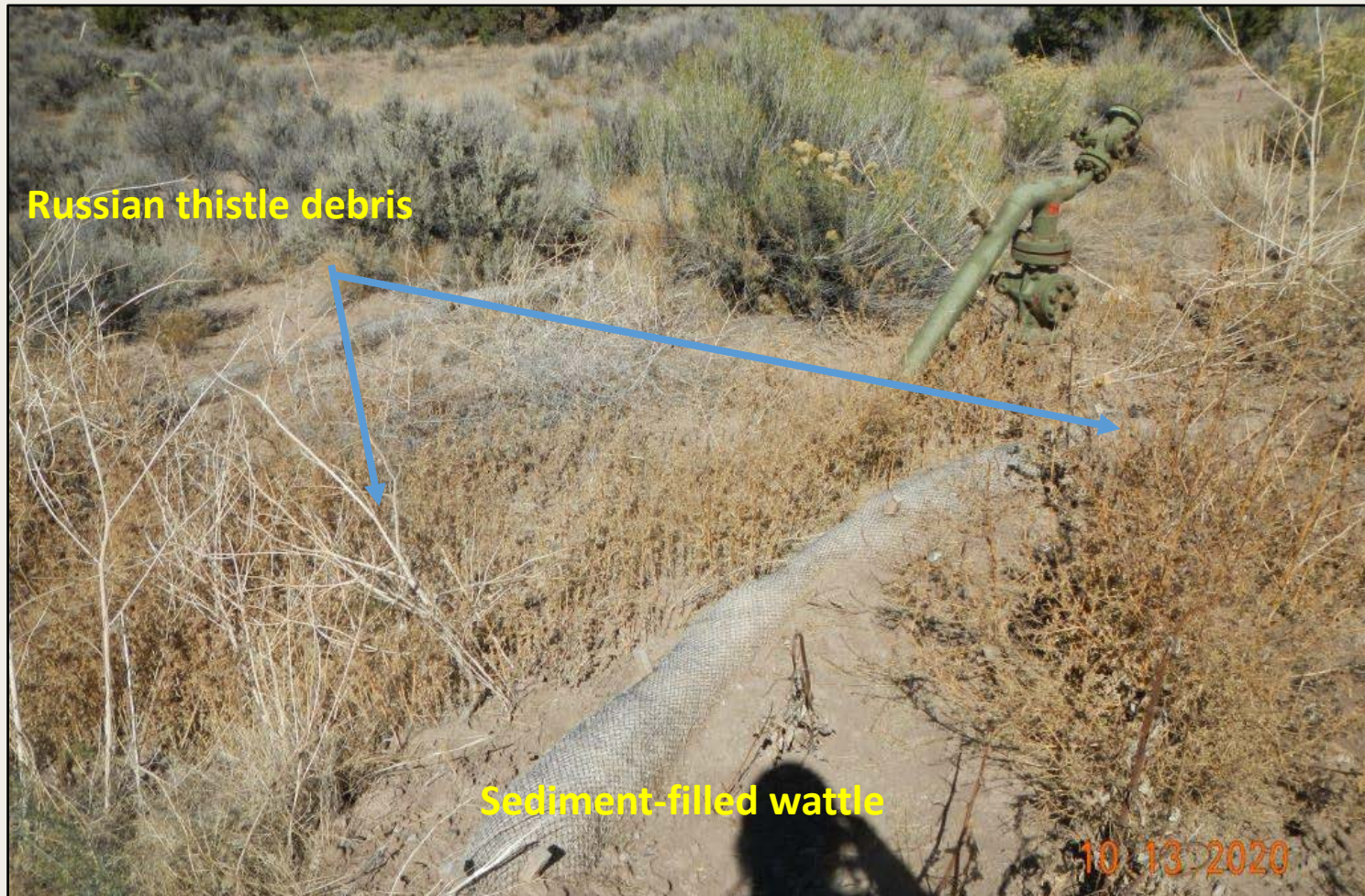
Photo 3. View of stormwater controls installed in the northern project area. The up-slope wattle is full of sediment and needs maintenance. Weed debris needs to be removed.
