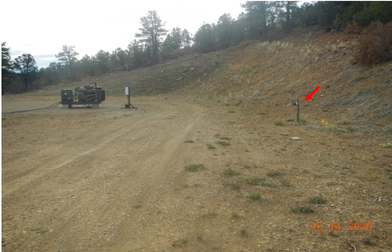
Photo 3. There is an unused riser which appears to be from the former meter shed of the CHAMPION #44-9 well.
