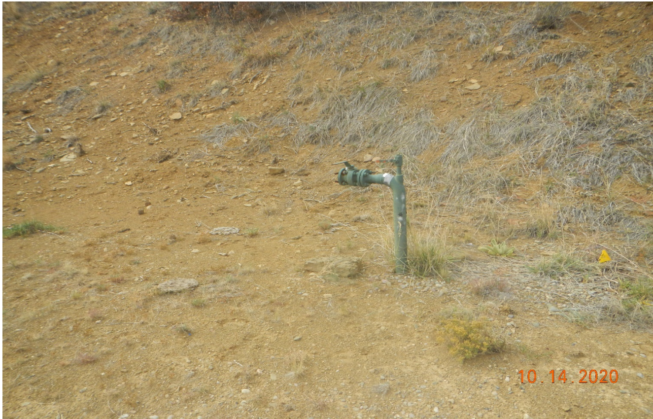
Photo 4. The unused pipe riser will need to be removed.
