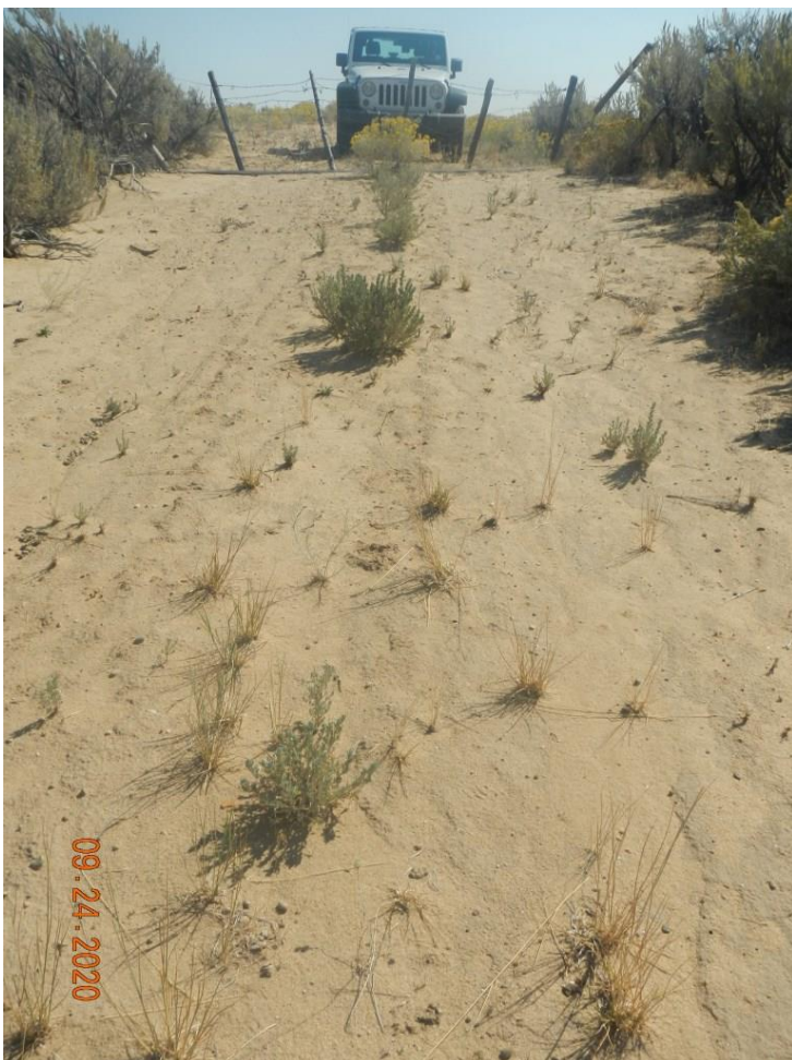
Photo#2: Portion of what was location road. Eroding sediment has washed over road burying vegetation.
