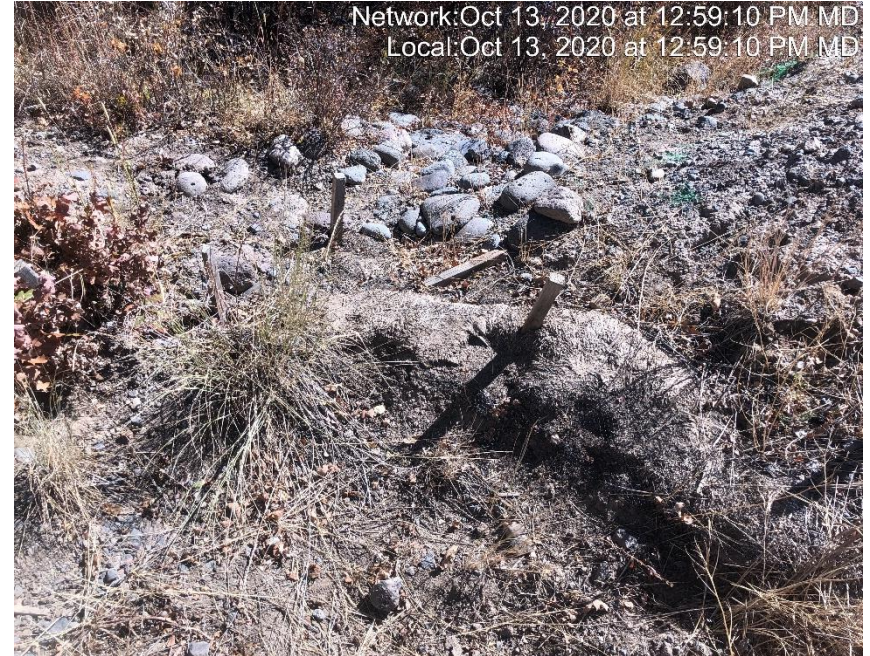
Photo #2011 Waddle in sediment trap has deteriorated and become debris.
