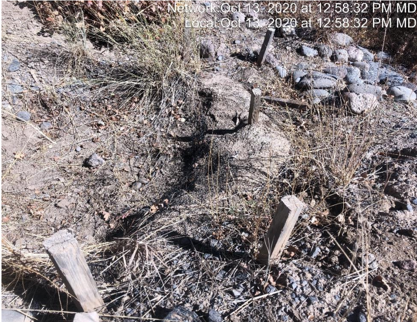
Photo #2010 Waddle in sediment trap has deteriorated and become debris.
