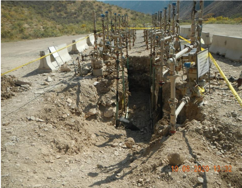
Excavation around wells exposing production flowlines.
