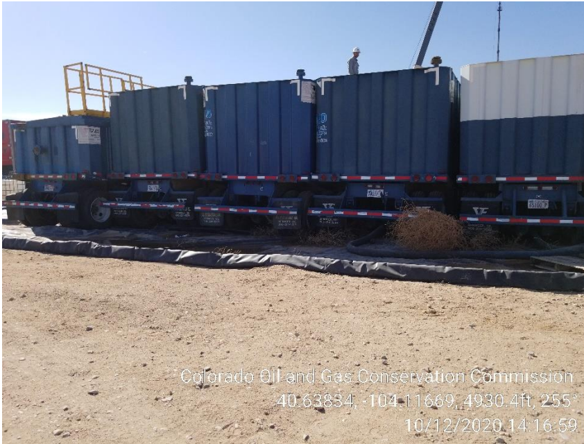
Photo 1 – Fresh Water Tanks not grounded
