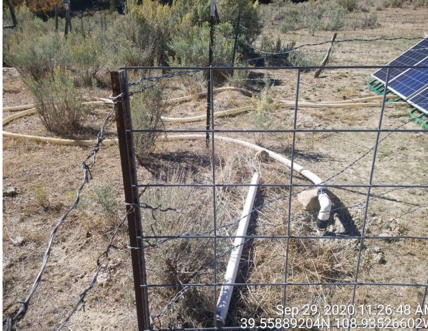
SVE well attached to the SVE system.
