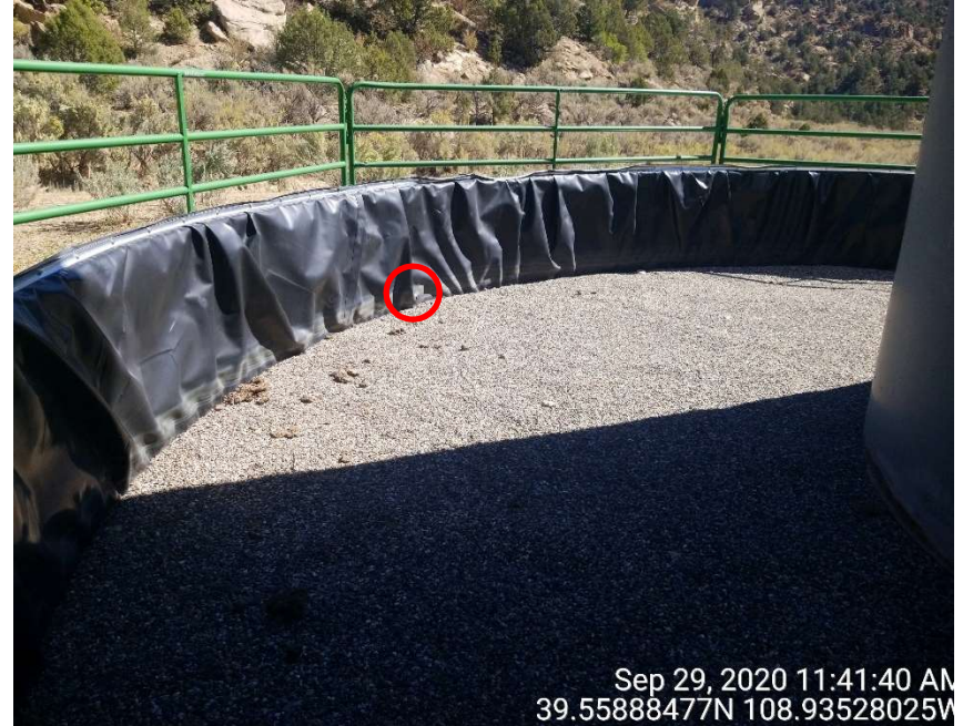
Hole in the tank battery secondary containment structure (red area).
