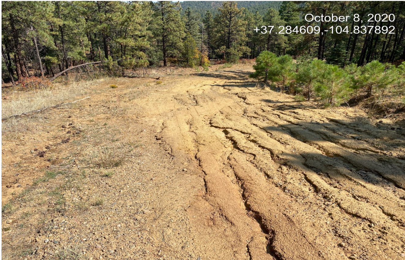
Photo 4. The access road has not been reclaimed and erosion is occurring.
