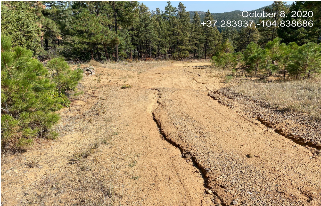
Photo 3. Facing west along the access road. Erosion is occurring along the road. Stormwater is flowing over water bars.
