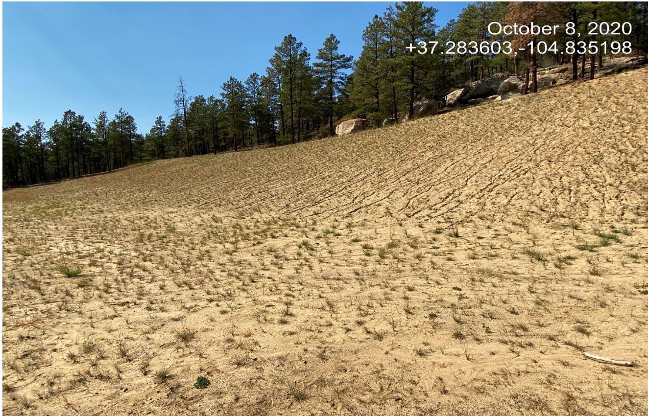
Photo 8. Facing southwest toward the location. The cut slope is not stabilized and there are signs of erosion.
