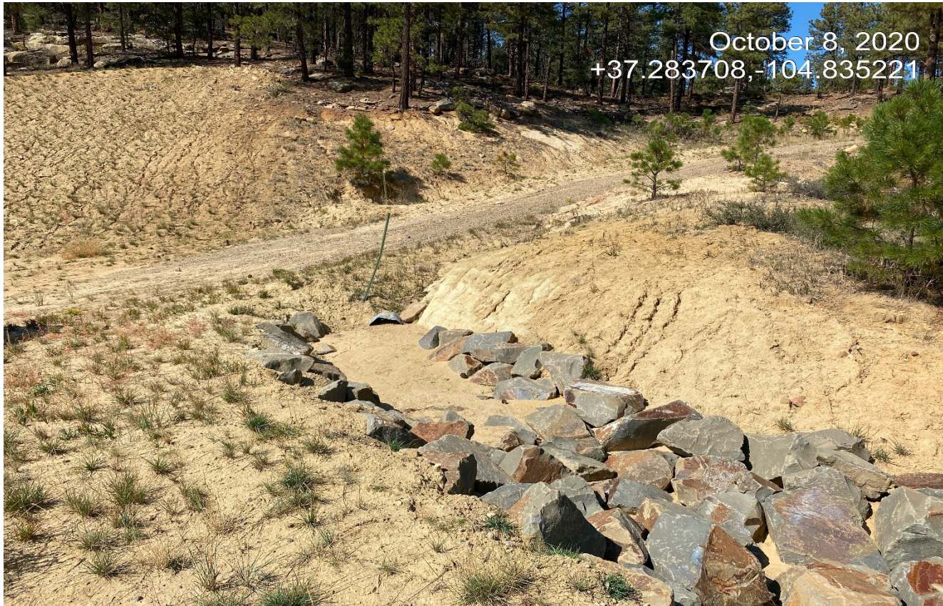
Photo 6. The culvert is filled in with sediment at the location. Culverts have not been removed.
