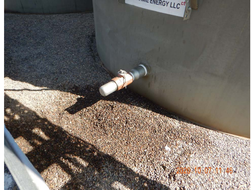
Photo #18 – Localized accumulation of oily waste beneath loadout for south tank.
