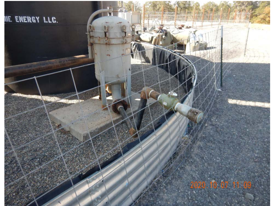
Photo #4 – Tank battery loadout with filter pot.
