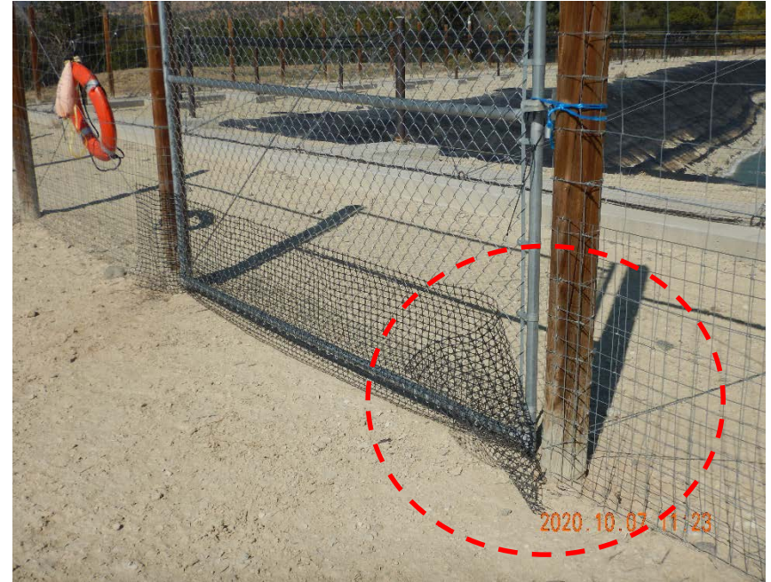
Photo #12 – Wildlife mesh was bent out on one side of south gate to pit on inspection date.
