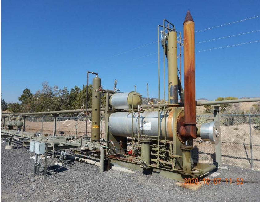
Photo #21 – Heated horizontal separator located along north side of compressor station.
