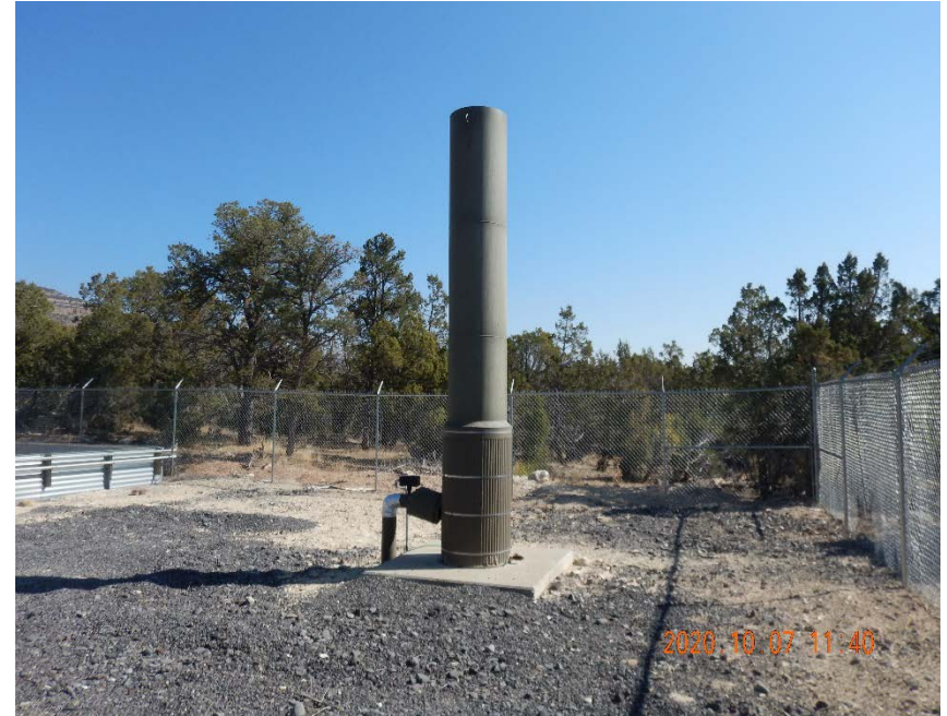
Photo #16 – Emission control device in southeast corner of compressor station.
