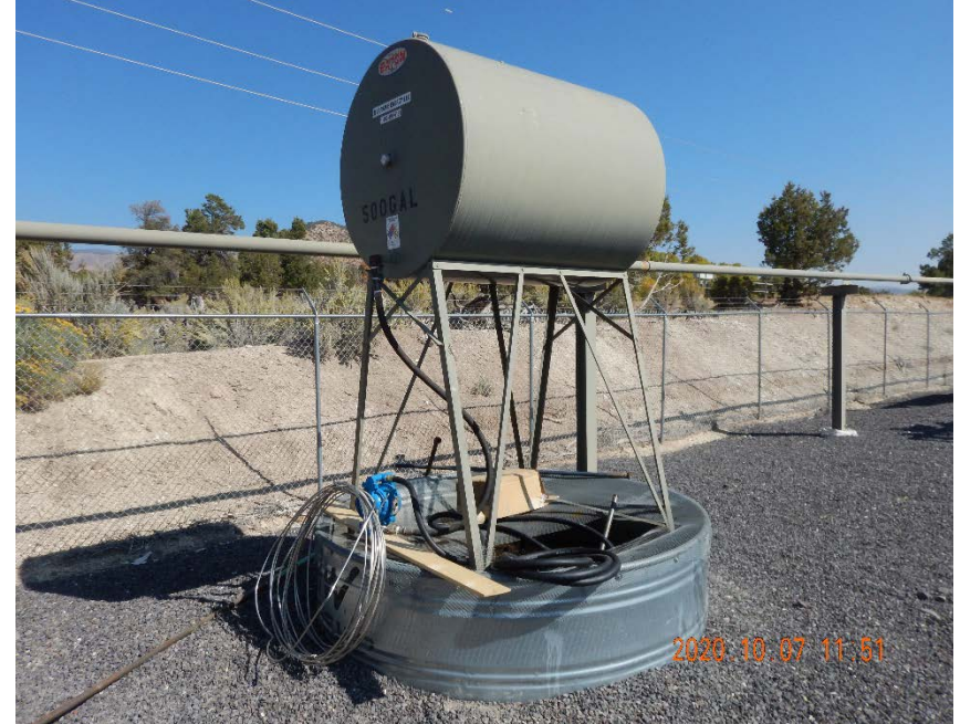
Photo #20 – View of 500 gallon N-triethylene glycol tank inside secondary containment located on north side of compressor station.
