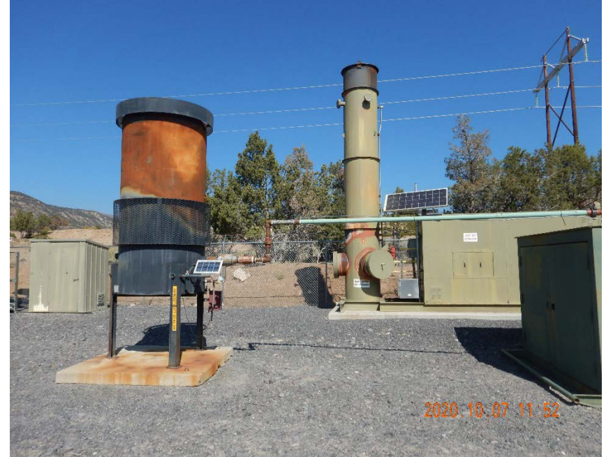
Photo #22 – Emission control device located in northwest corner of compressor station.
