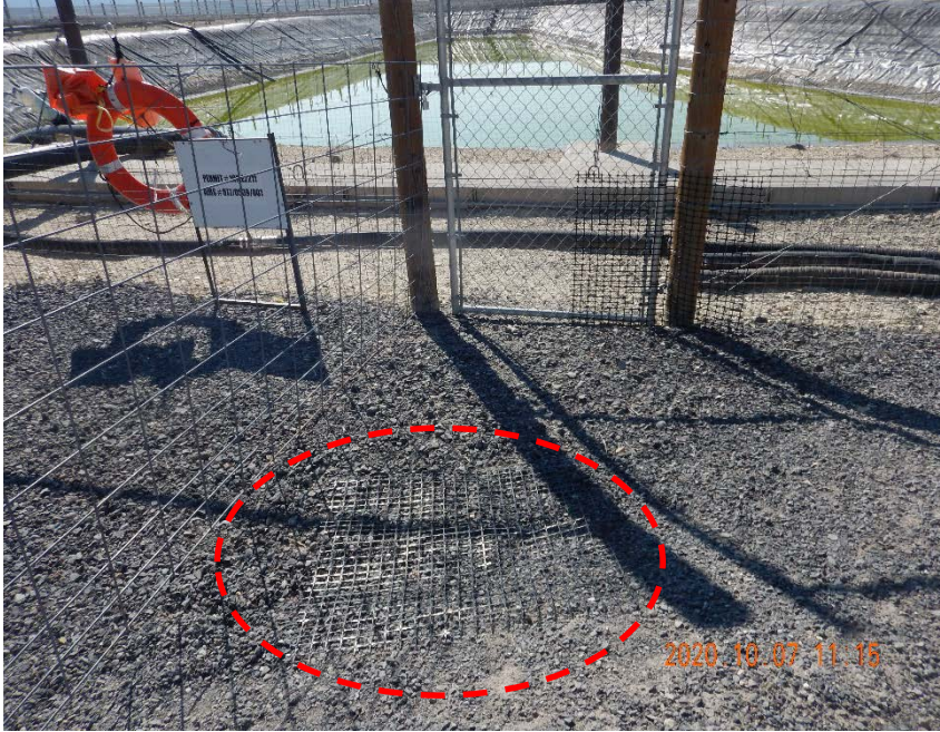
Photo #7 – Personnel gate on north side of pit. Note wildlife mesh is missing on one side. Red circle depicts location of mesh panel on ground.
