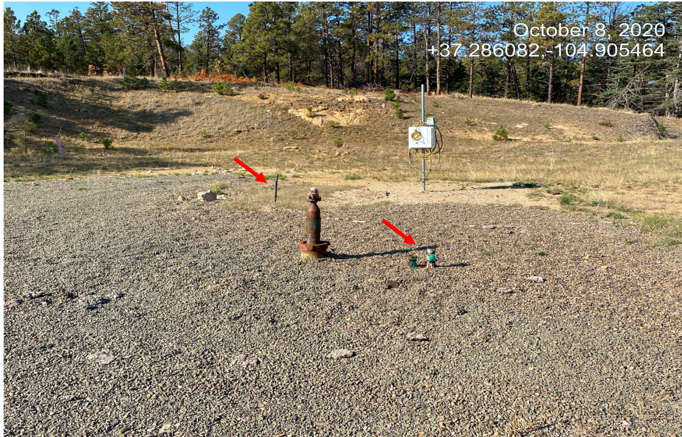
Photo 3. There is 3 unused risers that have not been removed per previous corrective action.
