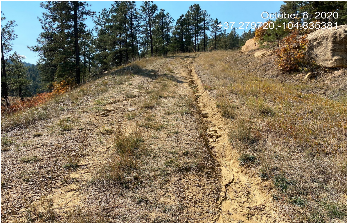
Photo 1. Facing southwest along the access road. There is erosion occurring down the road directed toward the county road.
