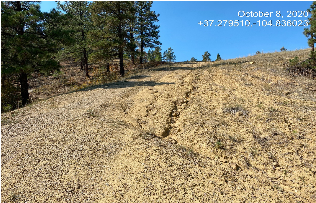
Photo 2. Facing west along the access road near the location. There is erosion occurring down the road.
