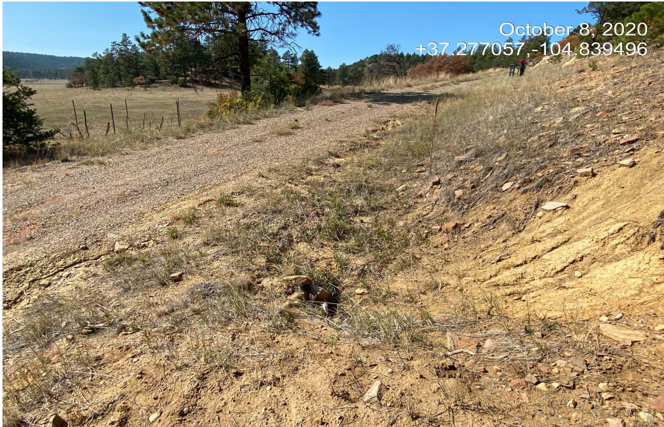
Photo 2. The culvert at the beginning of the road is filled in with sediment.
