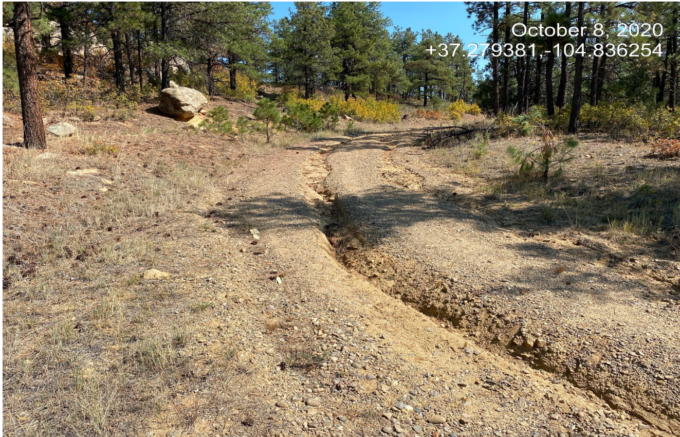
Photo 3. There is erosion occurring down the road. Stormwater is not properly diverted.
