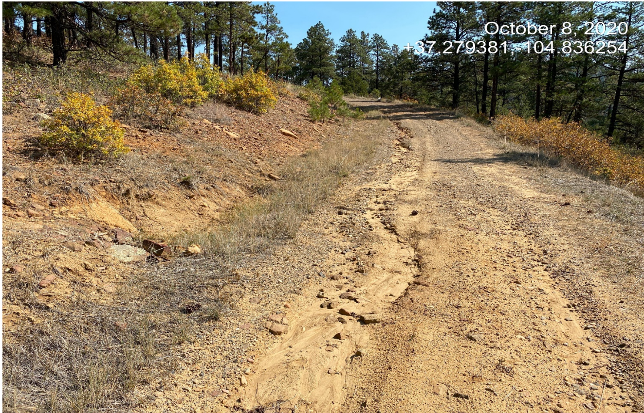
Photo 4. There is erosion occurring down the road. Stormwater is not properly diverted toward the culvert. Culvert is filled in with sediment.
