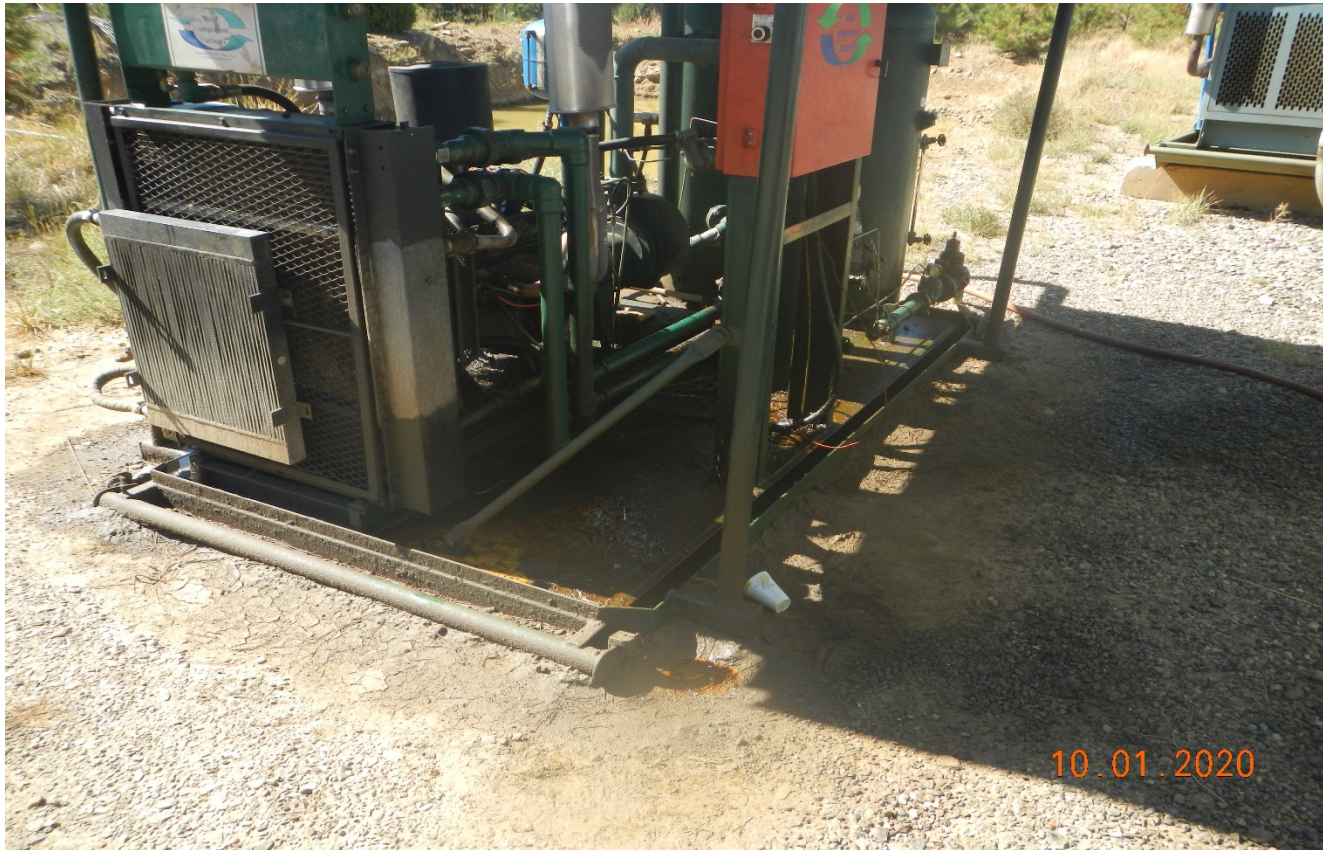
Photo 5. There is oily waste around and in the engine skid.
