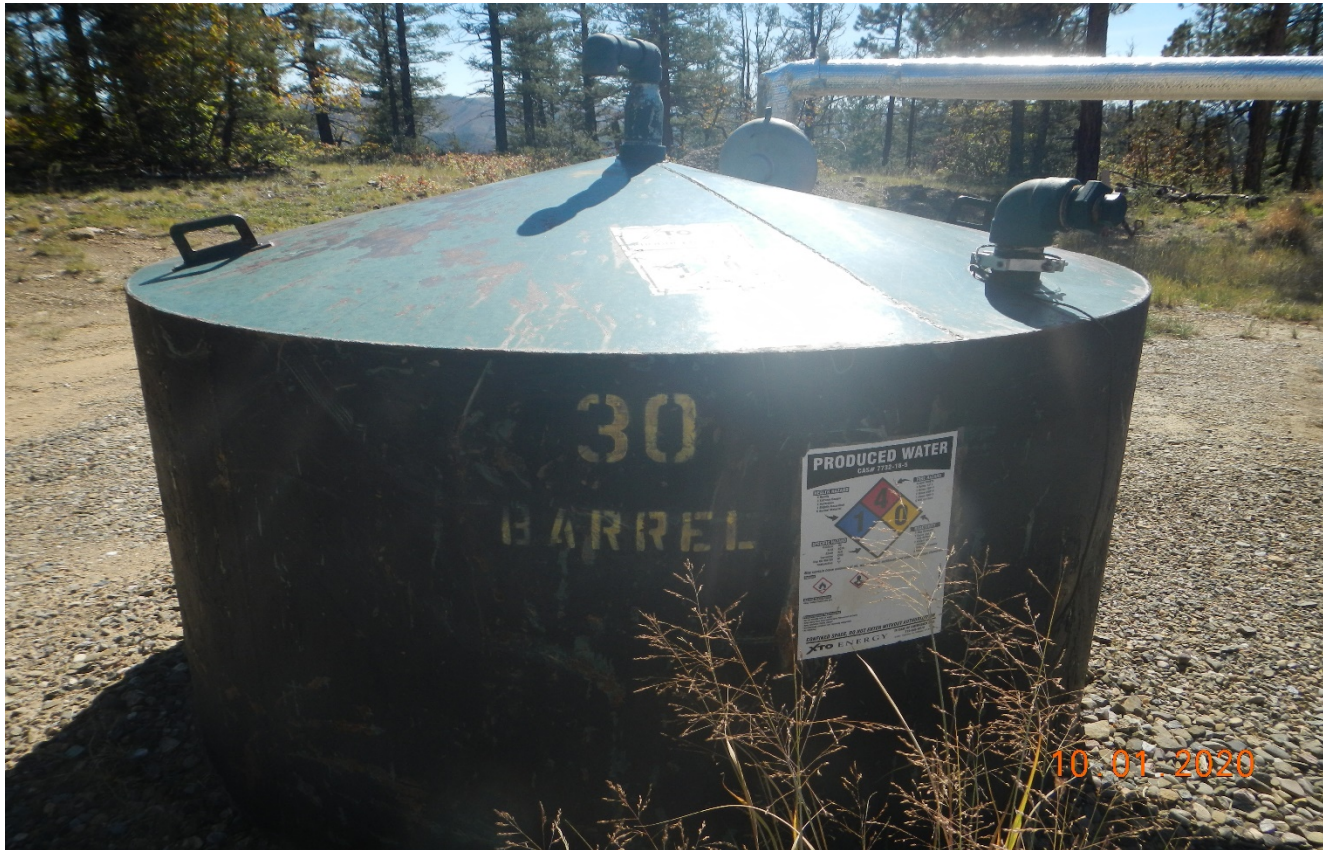
Photo 3. 30 Barrel produced water tank.
