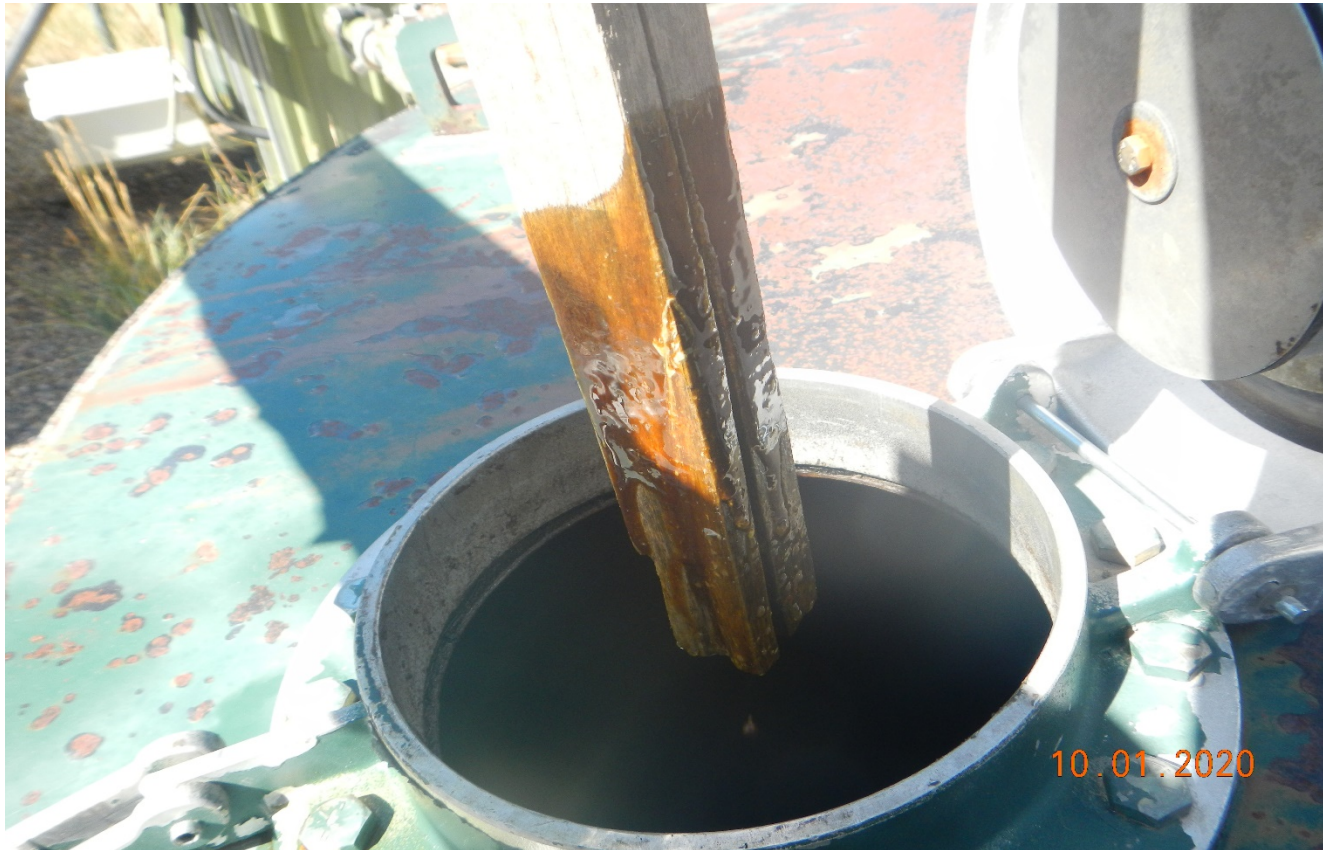
Photo 4. There is oil inside of produced water tank which is estimated to be 1/3 full. The hatch of the tank was opened and a stick was used to observe the liquid in the tank which shows the presence of oil inside of tank.
