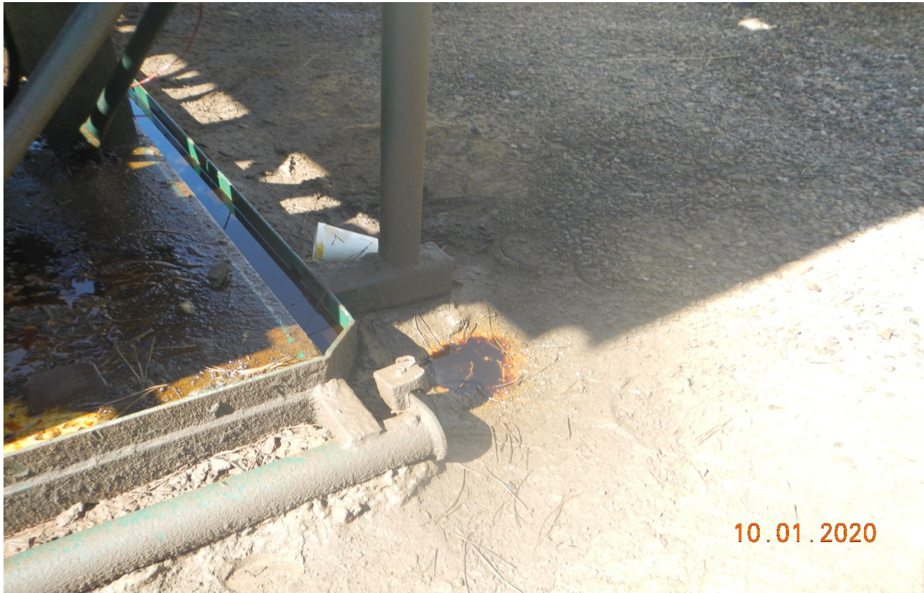
Photo 6. The engine skid is full of oil and there is saturated oil on the surface.
