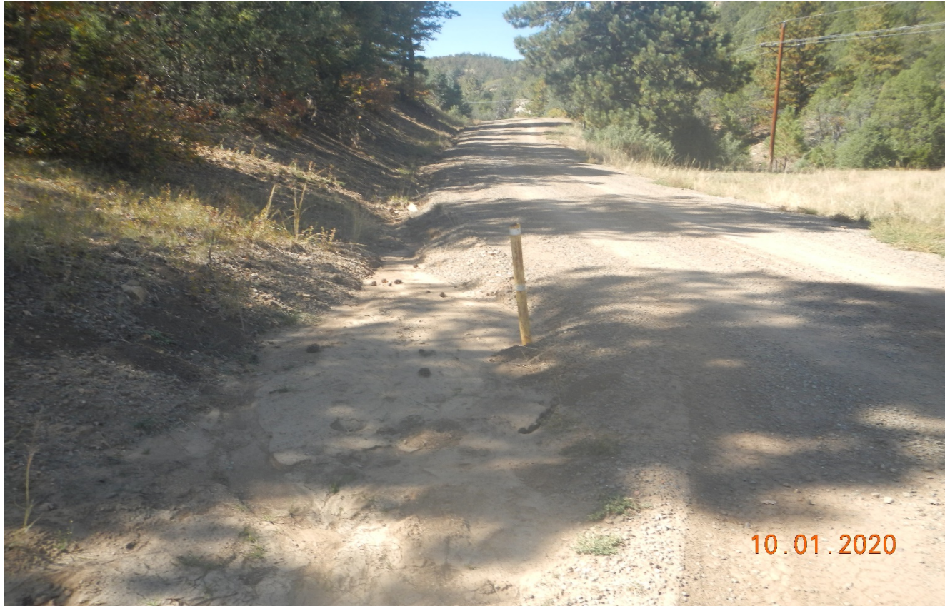
Photo 2. The culvert is filled in with sediment causing stormwater to flow down the road. All culverts need to be maintained. Previous corrective action was not performed.
