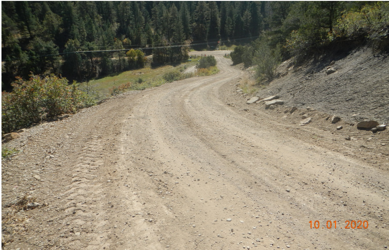
Photo 4. Facing back down the road which has been regraded. This area will need additional BMP's along the road side yo prevent erosion.
