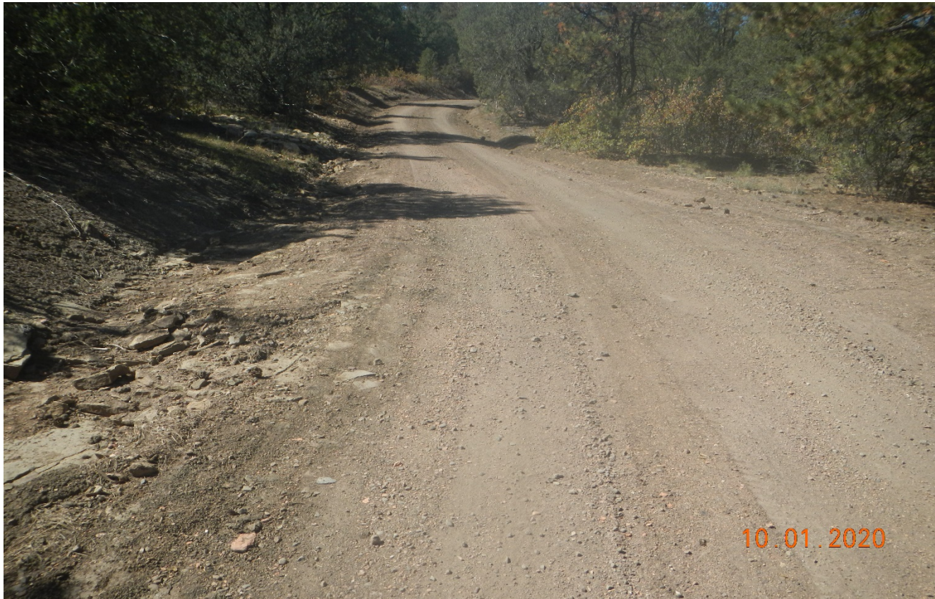
Photo 5. Facing northwest along the access road. The road has been graded and erosion along the road is repaired.
