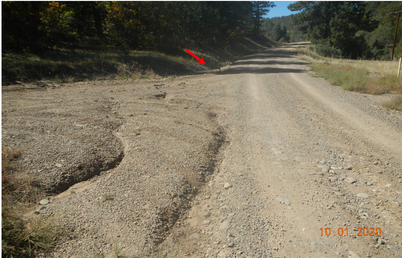
Photo 2. There is a plugged culvert along the main road (red arrow) causing stormwater to flow down the road. Lat/Long:37.09178,-104.93688. Corrective action was not completed.
