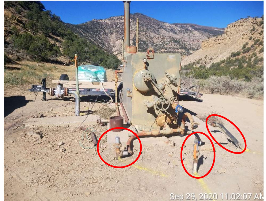
Separator, note the unmarked risers (red areas).
