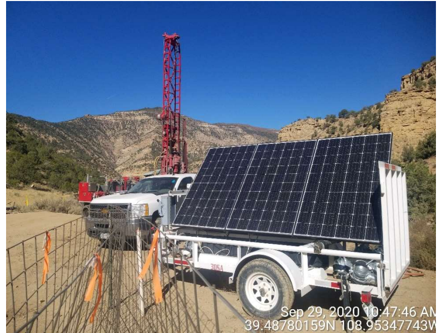
Monitoring well drill rig and solar powered SVE system.
