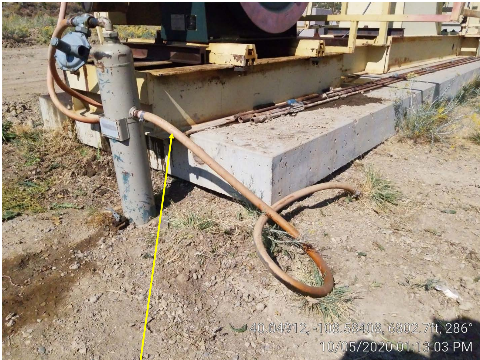
Photo 6. Hose leaking gas.
