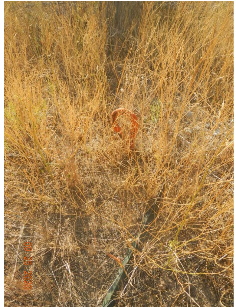
Photo#7: Anchors have not been removed.
