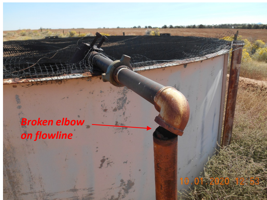
Close up of Broken elbow on flowline.
