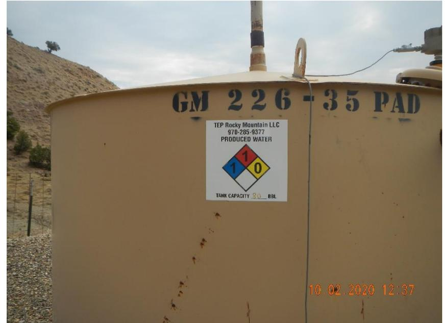
**Capacity on tank label is too small/faint to read from a distance.**
