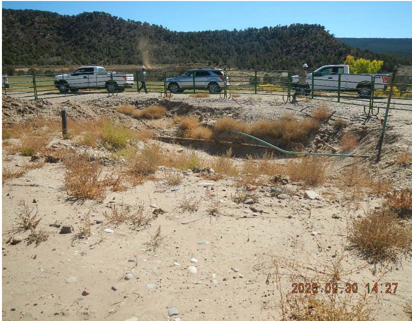
Evidence of surface water run on into excavation.
