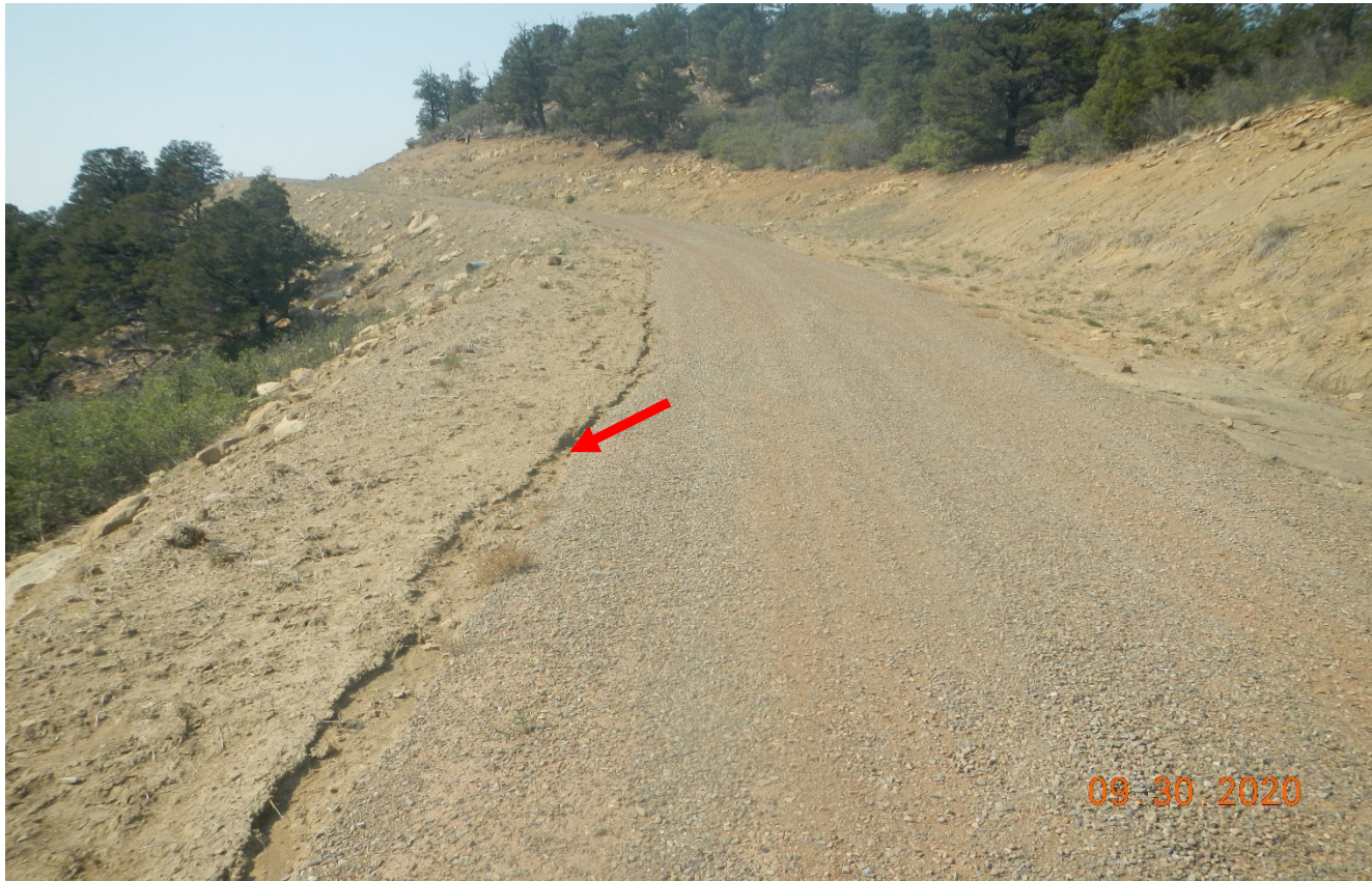
Photo 9. There is erosion beginning to channelize along the road which will worsen if not repaired.
