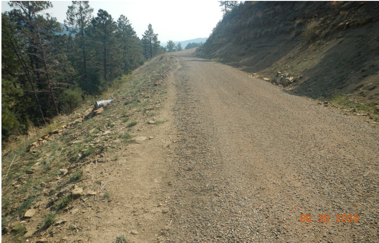
Photo 2. Facing southeast along the road. A culvert has been installed along this area of the road where the soil slough had occurred.
