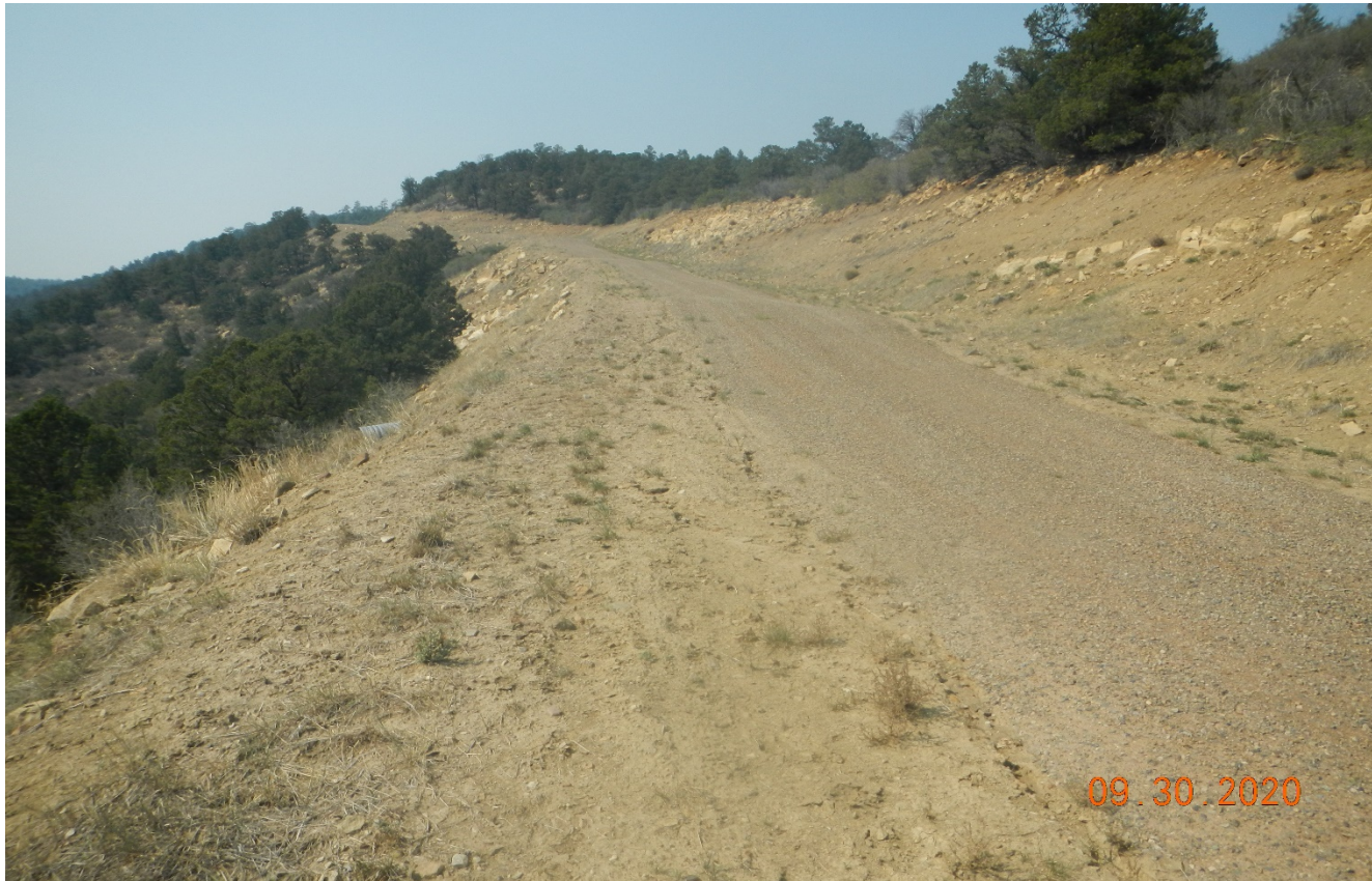
Photo 8. Facing northwest along the access road ascending the hillside. Gravel has been installed along the road. The roadsides will need to establish vegetation for stabilization.
