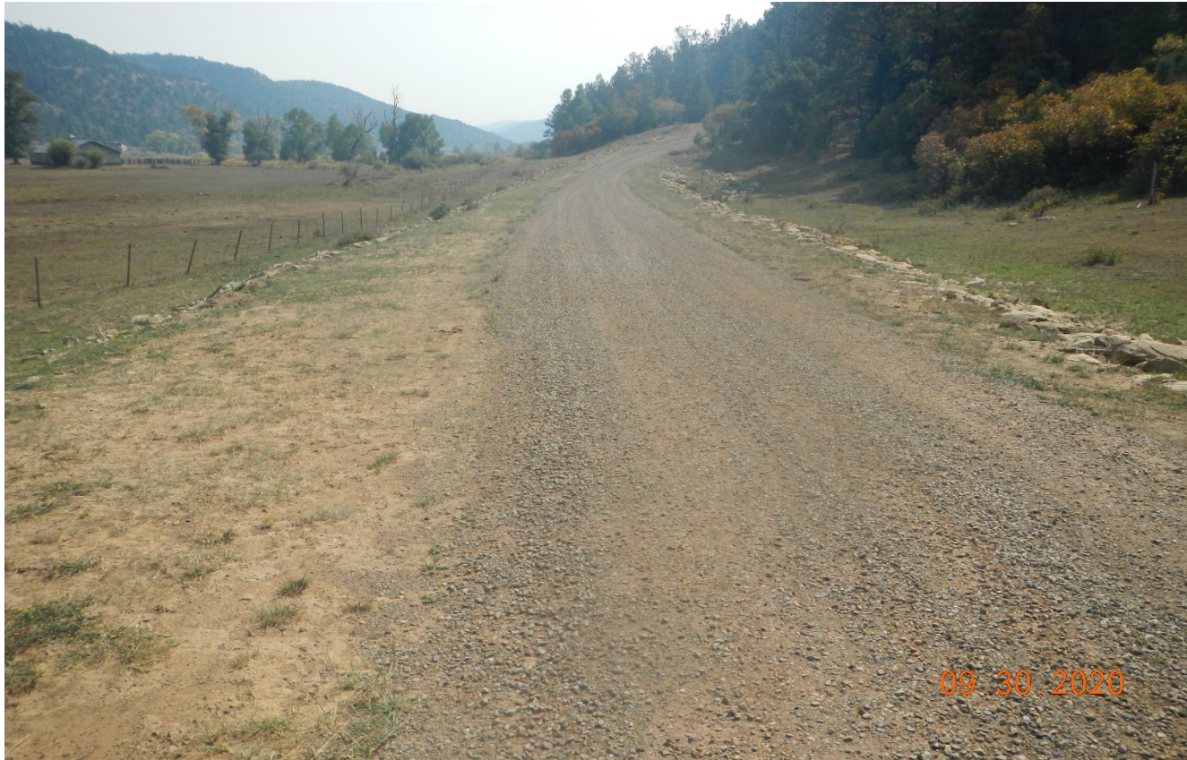
Photo 1. Facing southeast along the access road. The road all the way to the location has been graveled.
