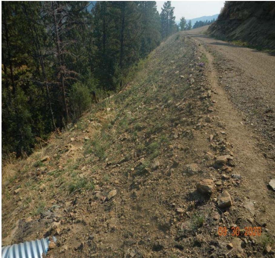
Photo 3. The photo on the left shows the area that was repaired from the slough that occurred in 2017 shown in right photo.
