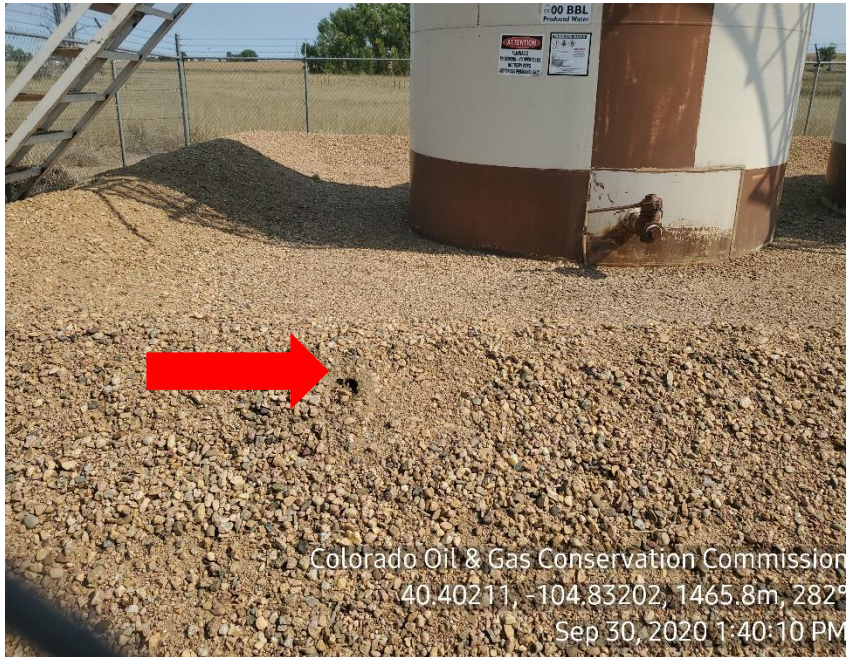
Photo 5: Hole in berm wall
