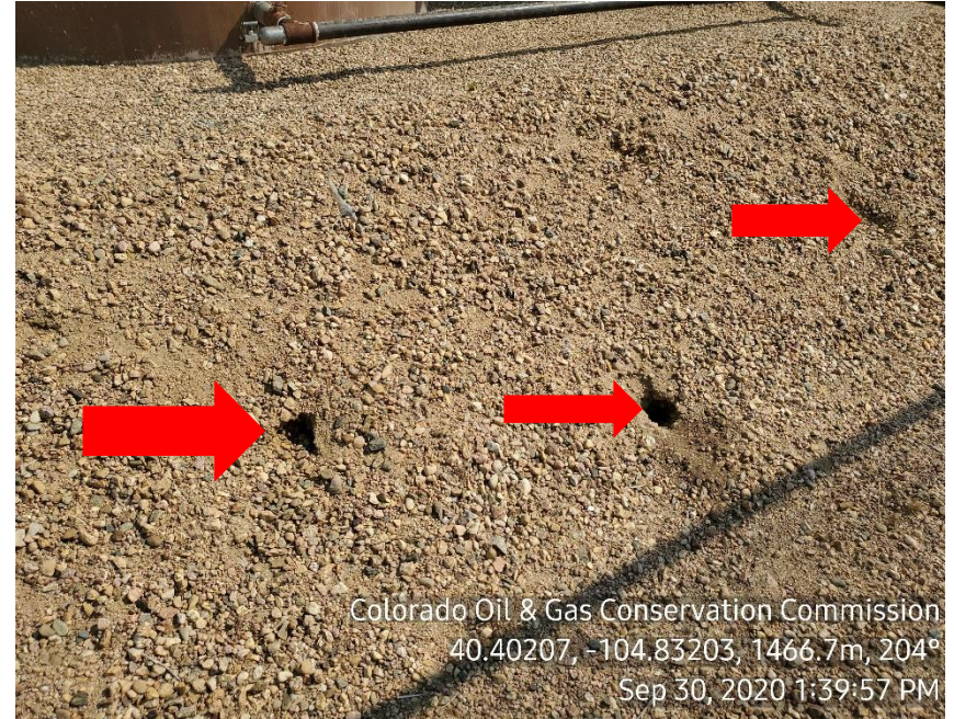
Photo 4: Holes in berm wall
