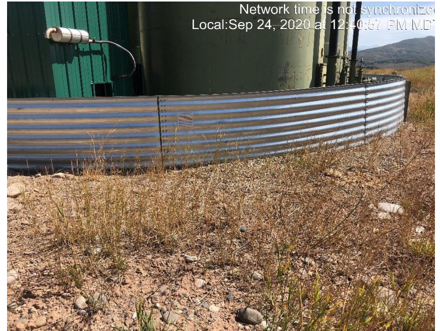
Photo #1920 Multiple places with debris encroaching on tank containments.
