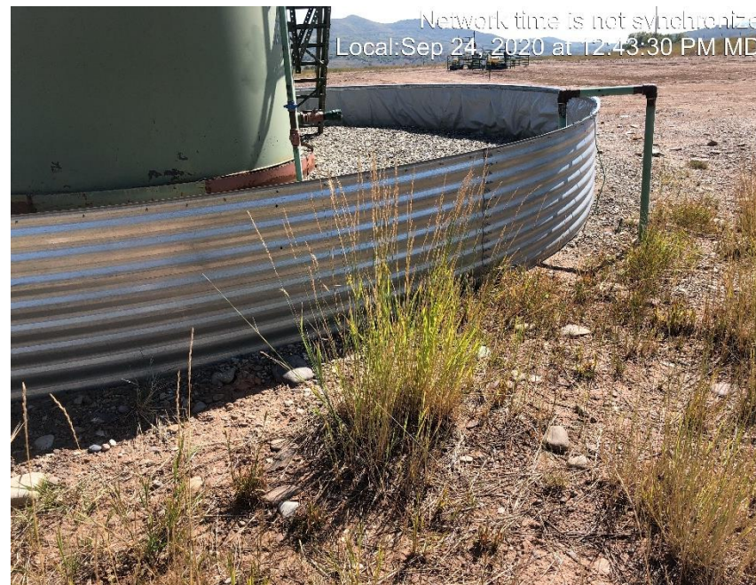
Photo #1924 Multiple places with debris encroaching on tank containments.
