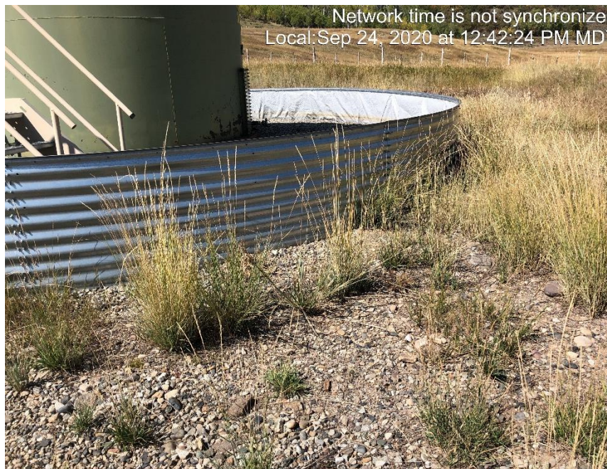
Photo #1923 Multiple places with debris encroaching on tank containments.
