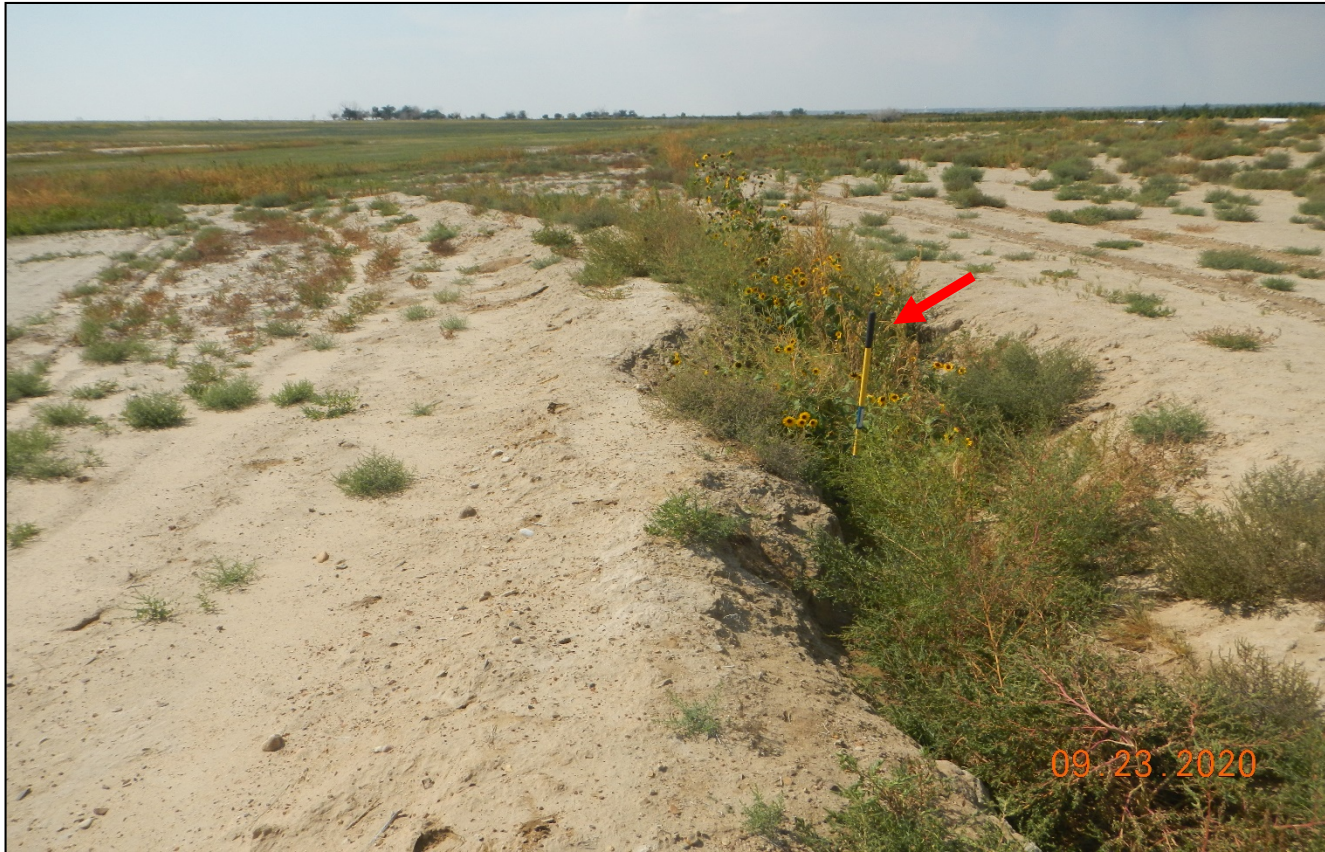
Photo 3. The diversion ditch at the north side of the location has not been recontoured. Arrow points to 4.5 ft. shovel placed in ditch.
