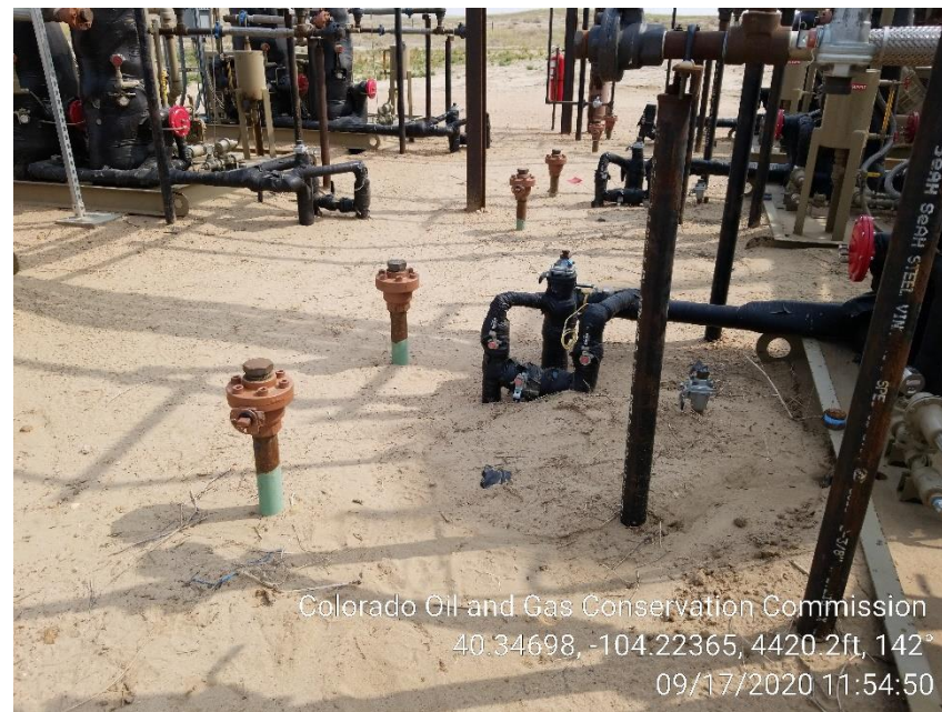
Photo 10 – Unmarked Risers at VRUs
