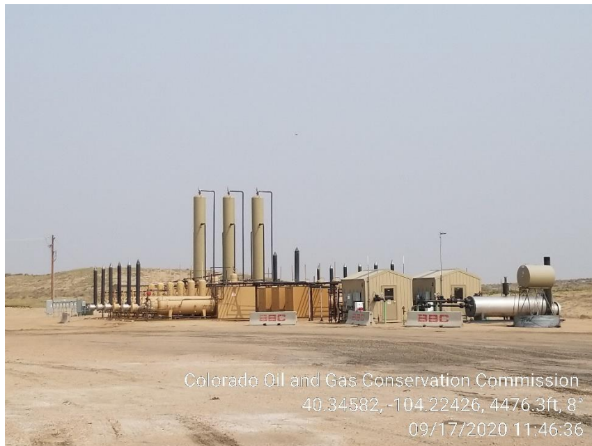
Photo 7 – Separators, VRTs, Gas Meters
