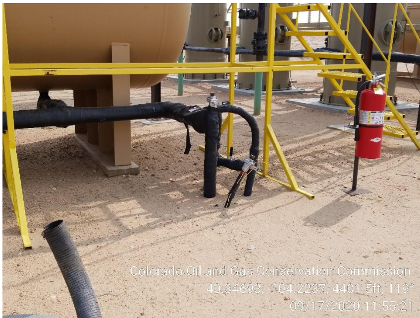
Photo 11 – Unmarked Risers at Horizontal Separator
