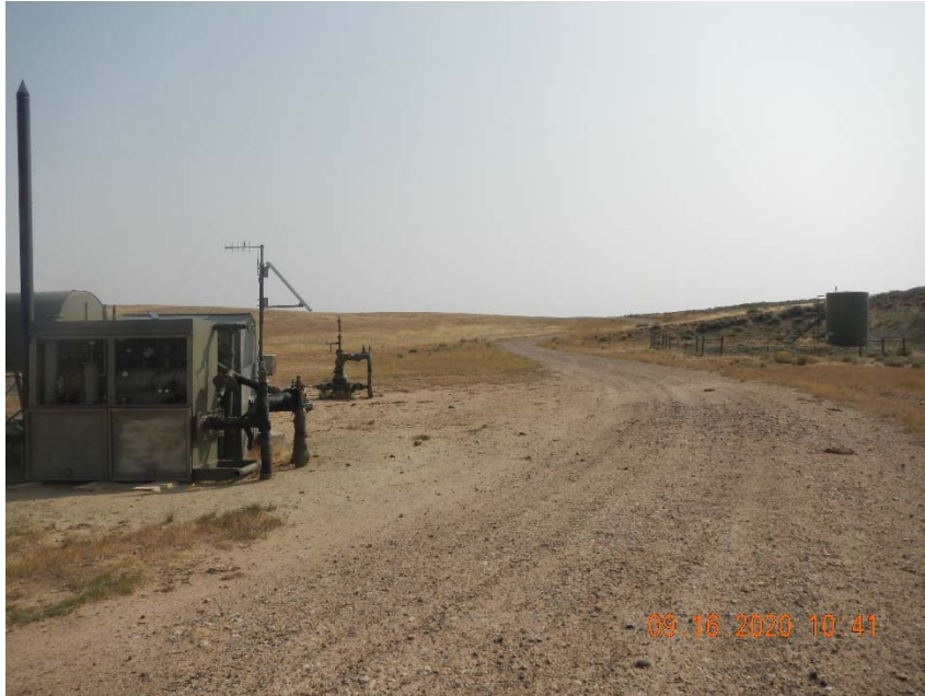
Photo 1. Overview of location taken facing east. Separator does not appear operable.
