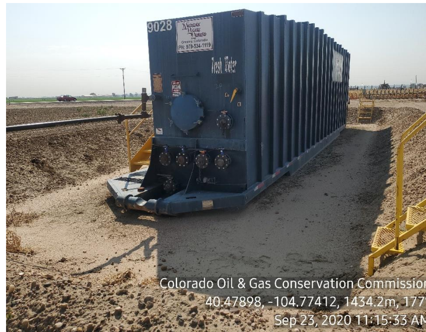
Photo 2: Tank not grounded
