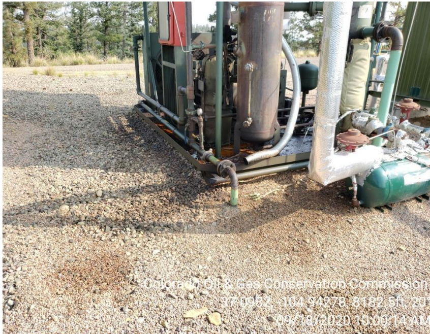
Photo 3 Stained soil at liquid ring
