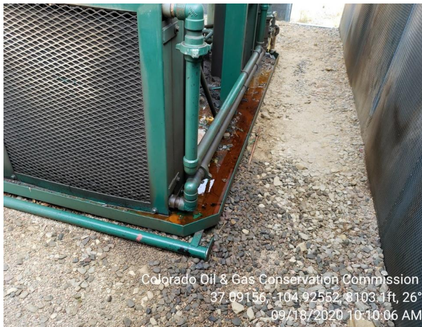
Photo 3 Stained soil at liquid ring
