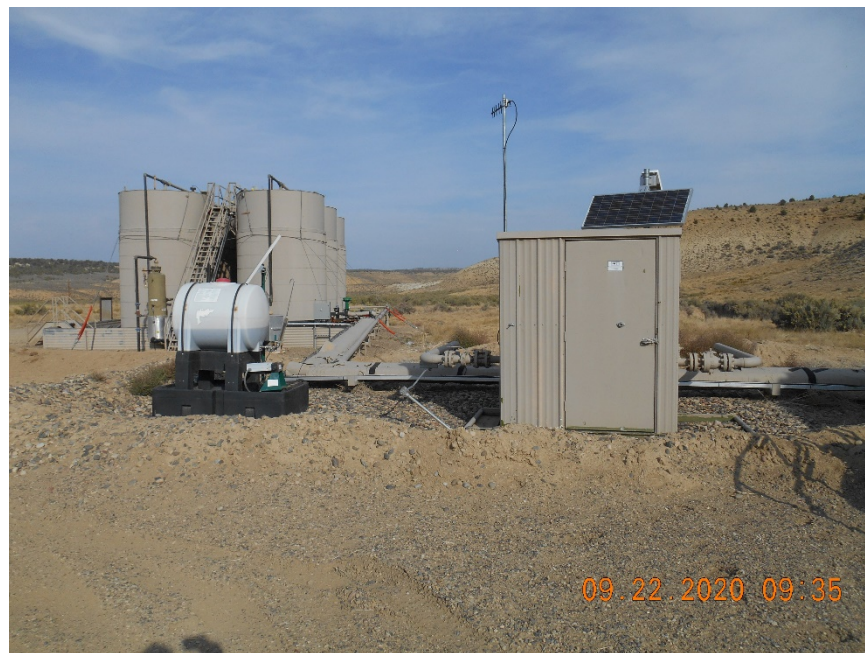
Meter Housing. Chemical containers with secondary containment.
