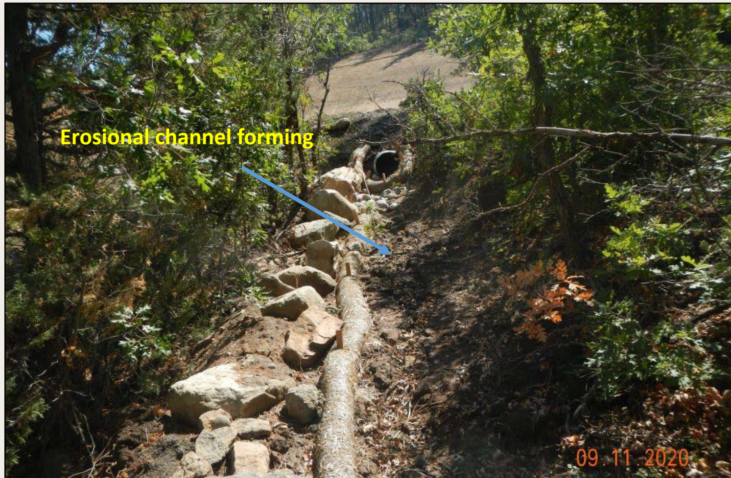
Photo 4. View of erosional downcutting occurring downstream from culvert outlet, near the well pad entrance. Wattle is placed along the slope.
