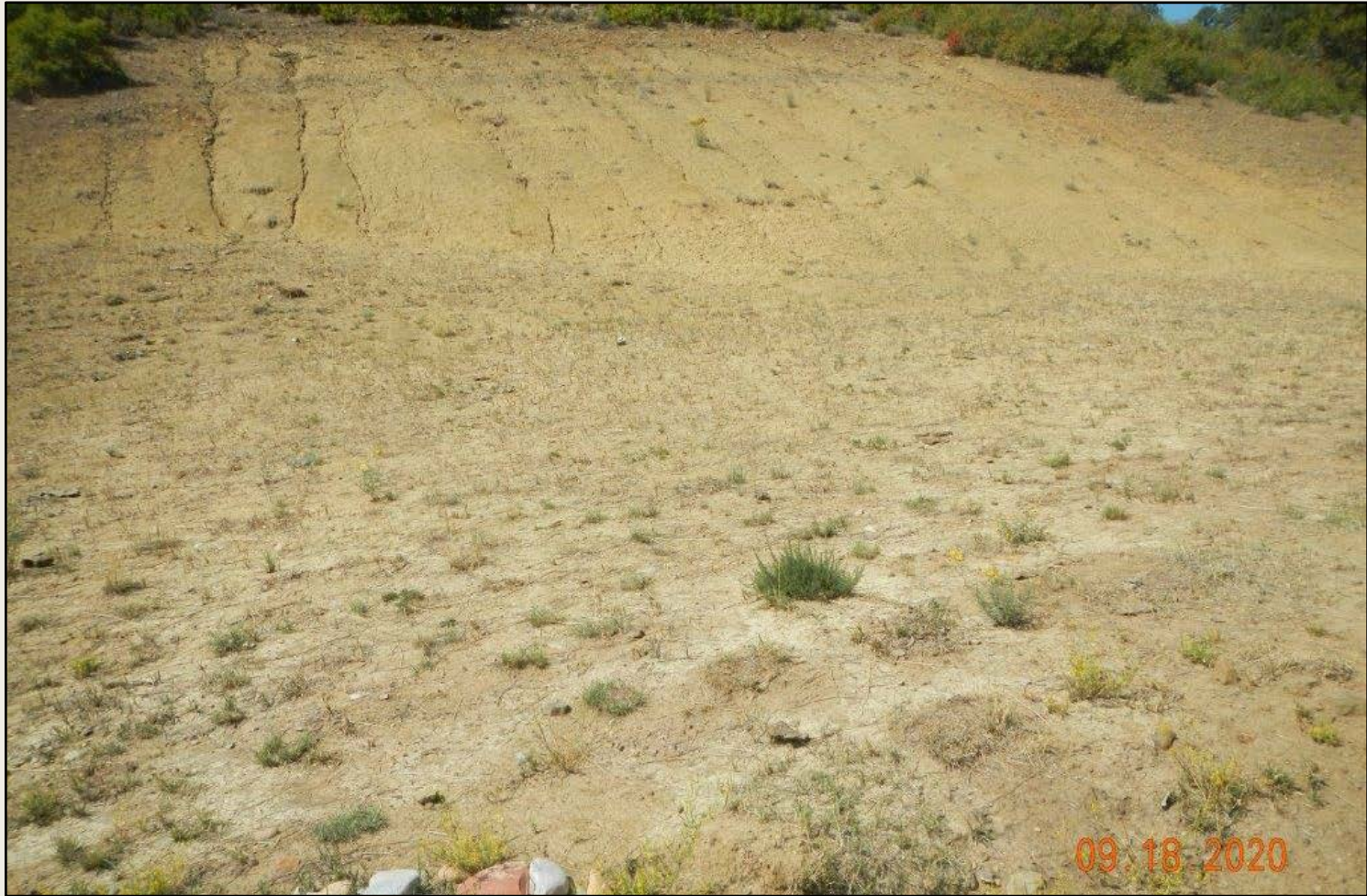
Photo 3. View of the western cut-slope showing areas that remain sparse and where additional stabilization is needed. Erosion controls need to be installed to stabilize erosion on bare soils until stabilized with desirable perennial vegetation.
