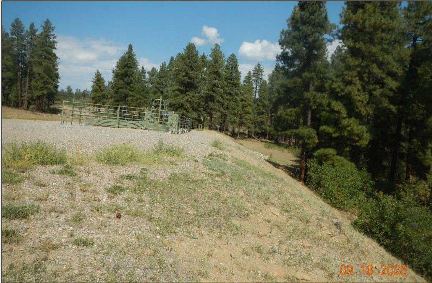
Photo 2. View of the eastern fill slope from the southeastern corner facing northward. Revegetation is progressing with grasses such as western wheatgrass and sand dropseed, largely in a grazed condition.
