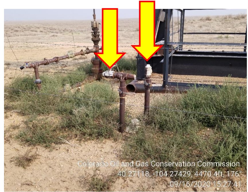
Photo 4 – Wellhead, Weeds, Unmarked Risers
