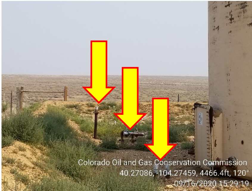
Photo 5 – Unmarked Risers and Weeds
