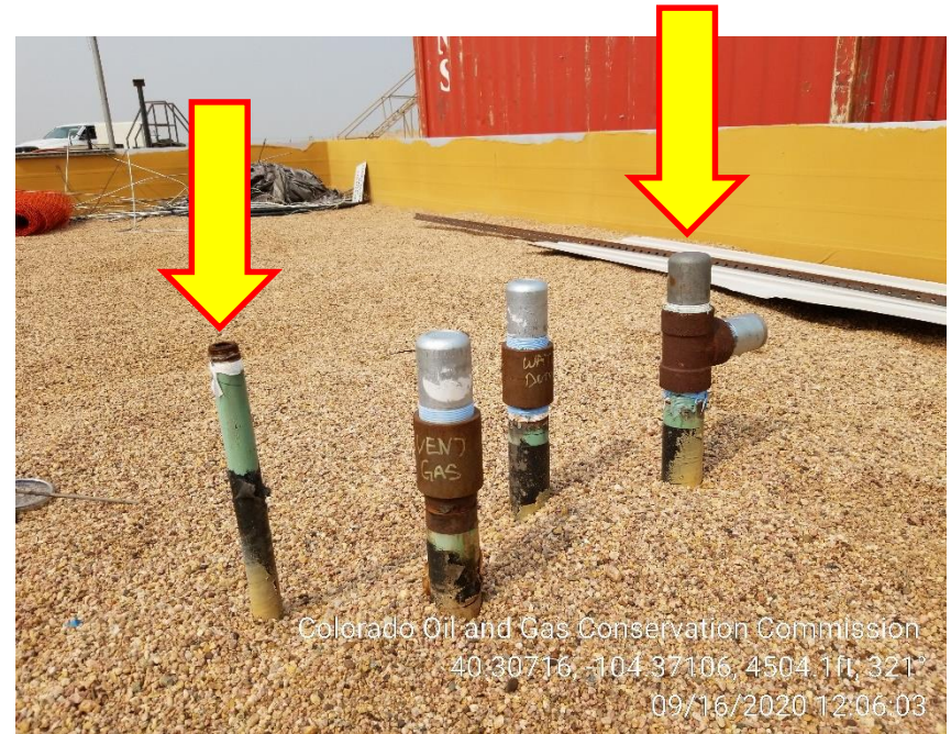
Photo 6 – Unmarked Riser where the old Separator was removed. Please mark ALL Risers
