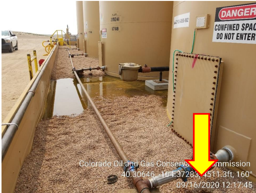
Photo 17 – Stained Soil at Drain Valves on NE Tank
