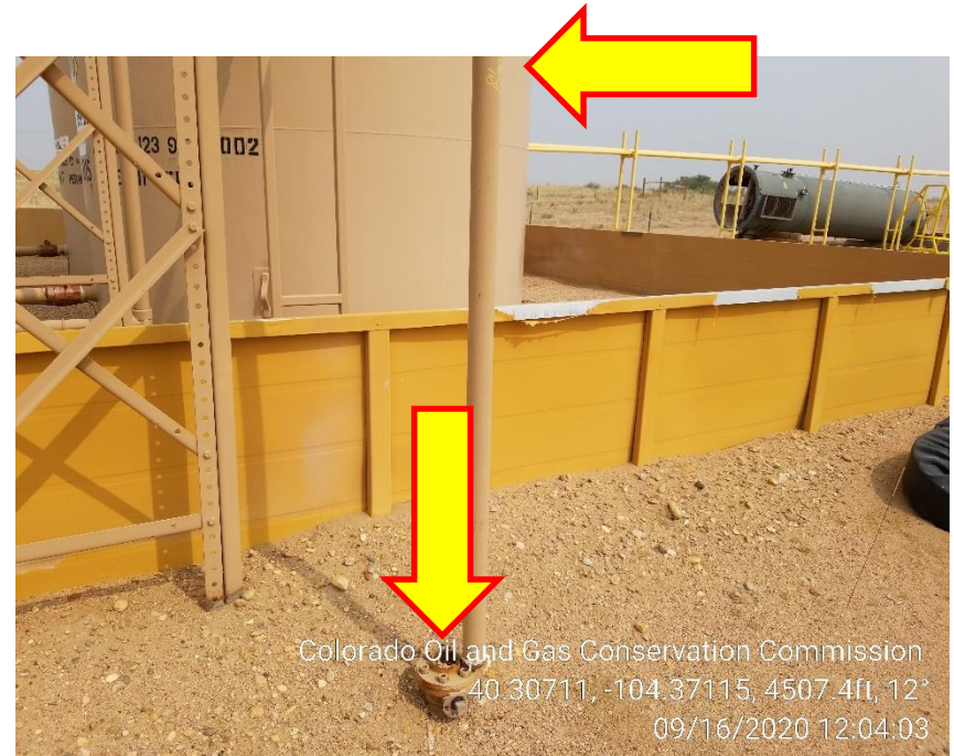
Photo 4 – Unmarked Riser at NE Tanks, Please mark the actual Valve coming up out of the ground as well.
