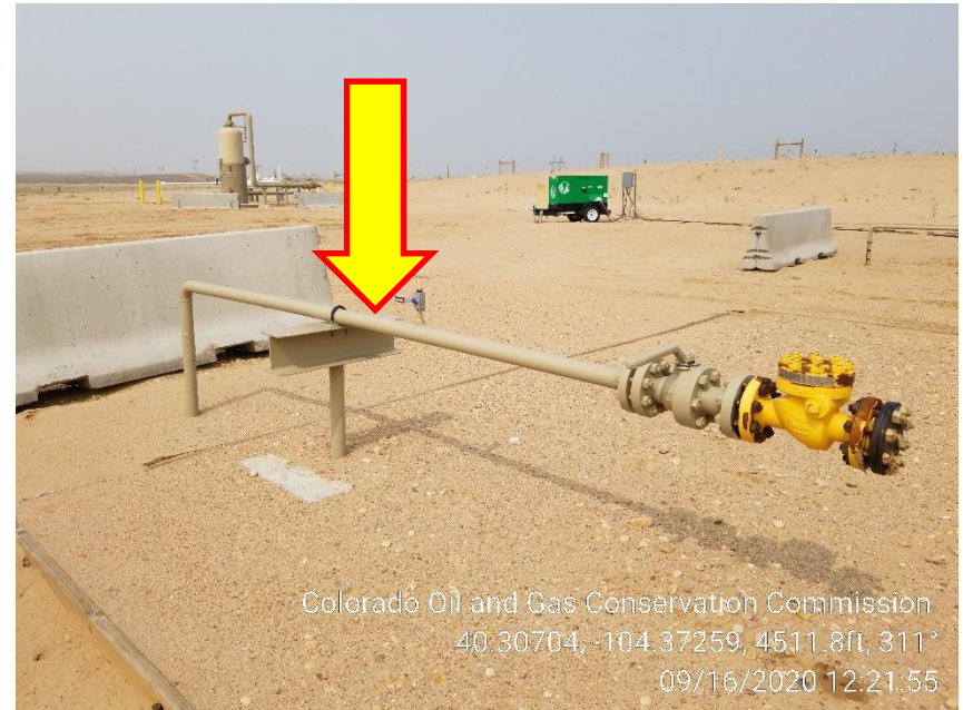
Photo 22 – Unmarked Riser at Compressor
