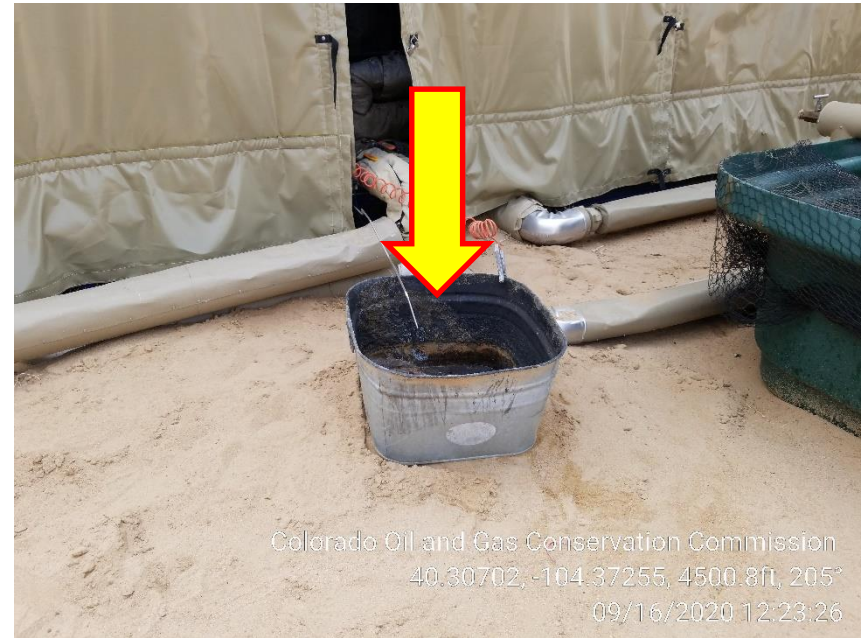
Photo 26 – Drain Bucket at Compressor missing Wildlife Netting
