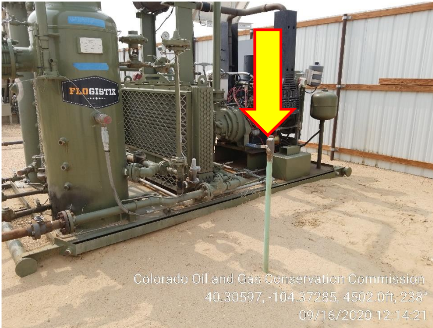
Photo 11 – Unmarked 1" Riser at VRU
