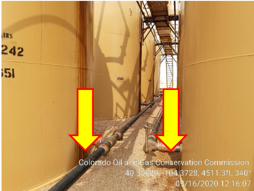
Photo 13 – Stained Soil at ALL Loadline Valves
