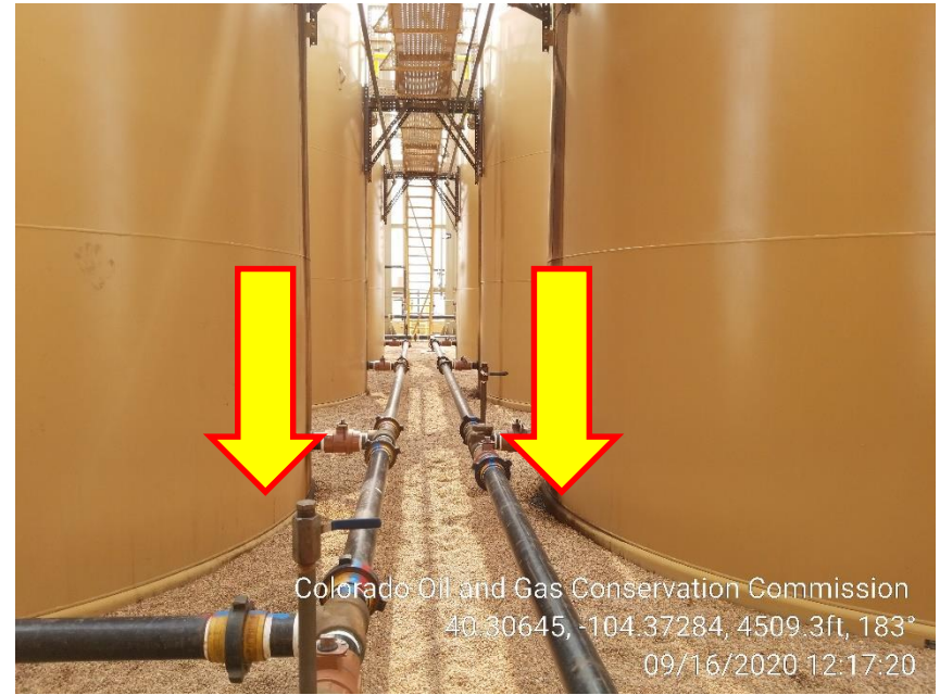
Photo 16 – Stained Soil at ALL Loadline Valves
