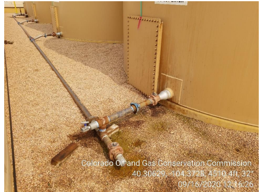
Photo 14 – Stained Soil at Drain Valves on SW Tank
