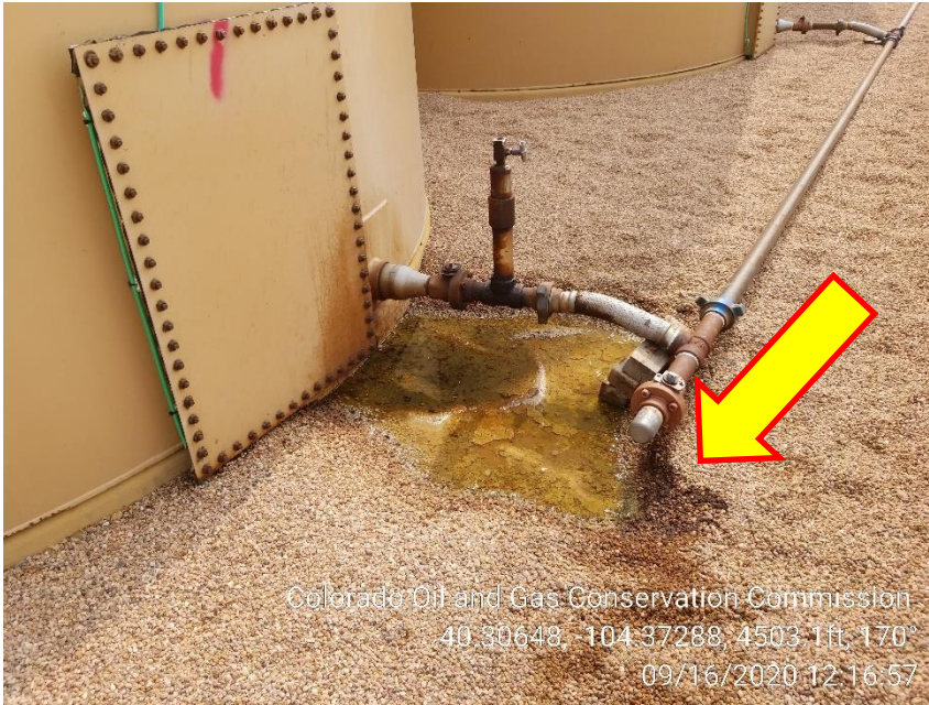
Photo 15 – Stained Soil at Drain Valves on NW Tank
