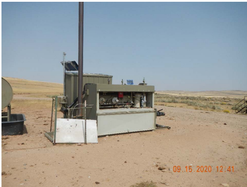
Photo 2. Separator does not appear operable.
