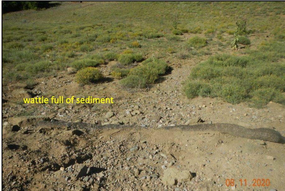
Photos 3/4. View of wattles in the western and southwestern project area that are full of sediment, displaced, and no longer functioning. Wattles are not adequate BMPs in these areas.
