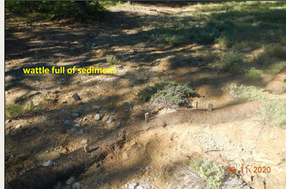
Photos 3/4. View of wattles in the western and southwestern project area that are full of sediment, displaced, and no longer functioning. Wattles are not adequate BMPs in these areas.
